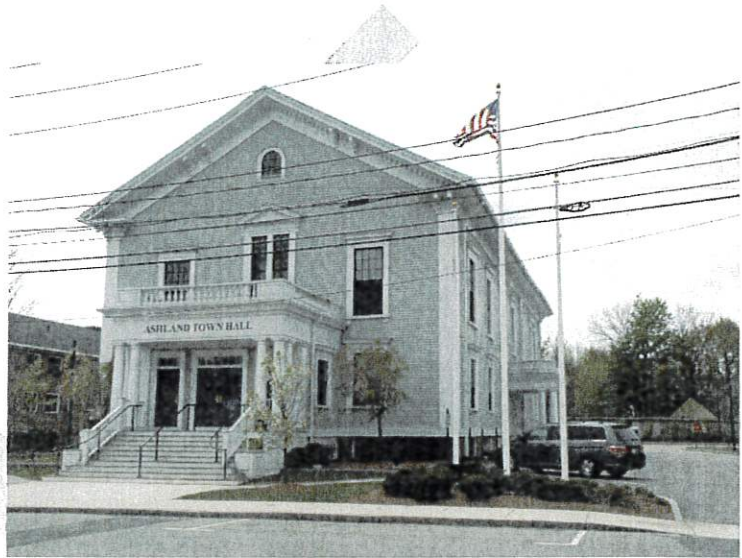
Ashland Town Hall Source: Town of Ashland Photo Gallery website
