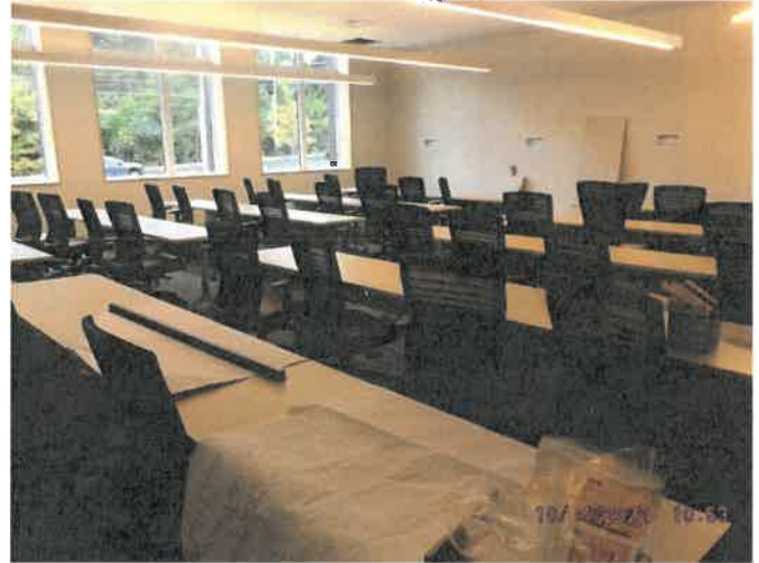
Photo depicts the progress of furniture install.
