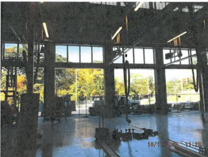
Photo depicts the progress of the apparatus bay doors.
