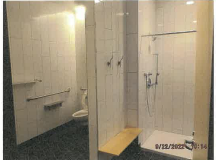
Photo depicts the substantially complete FD bathroom/shower.
