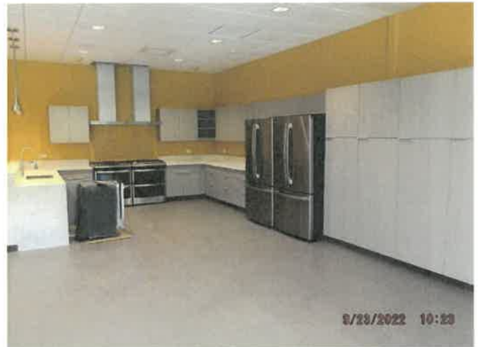
Photo depicts the progress of the FD kitchen.
