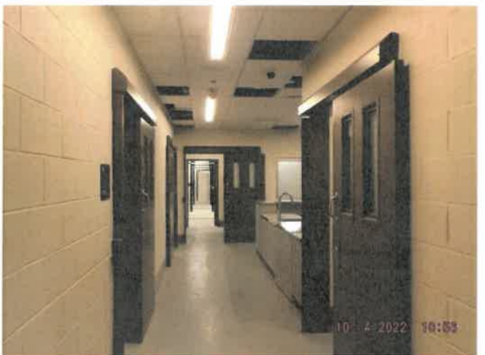
Photo depicts the substantially complete detention area.
