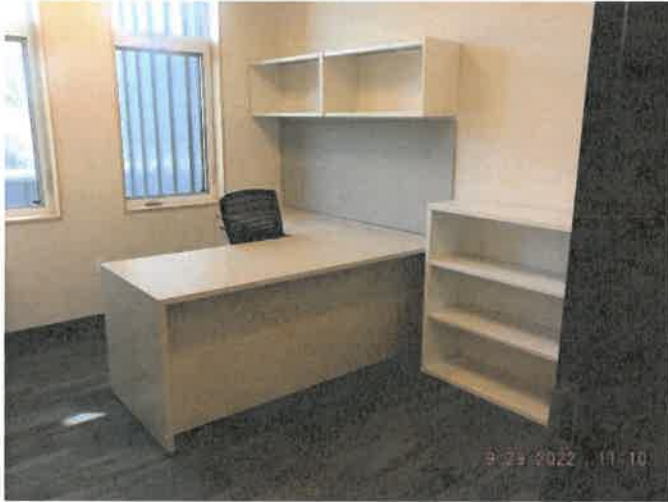
Photo depicts the progress of furniture installation
