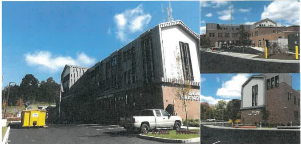
Pictures: Overall Site Progress
