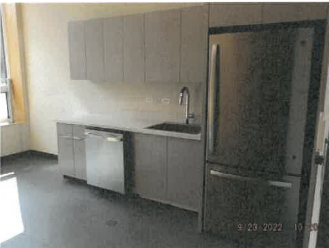
Photo depicts progress of the appliances
