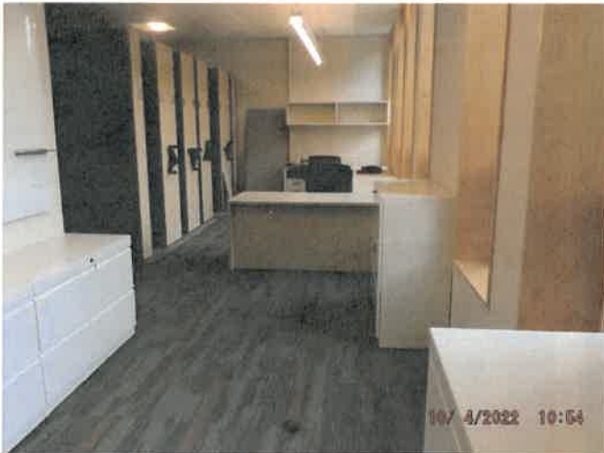
Photo depicts the progress of furniture installation.
