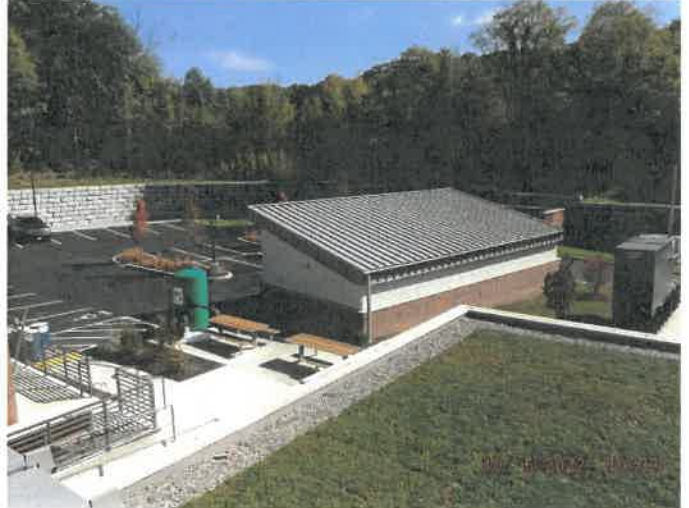
Photo depicts the substantially complete rear of site.
