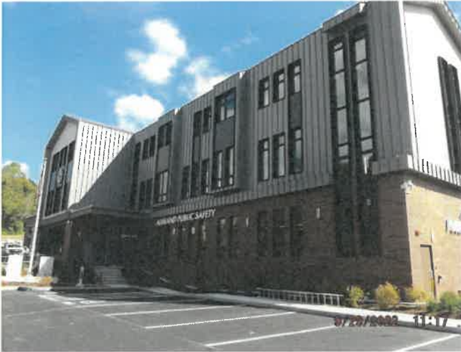
Photo depicts the substantially complete exterior.
