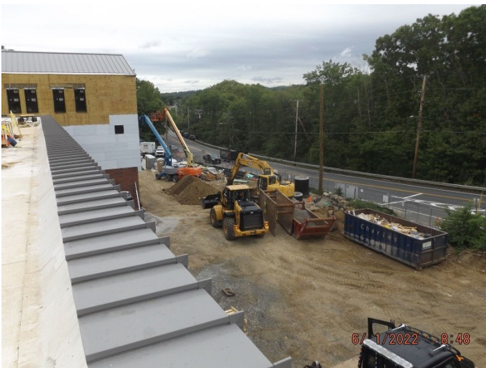
Photo depicts the progress of the front of the site.
