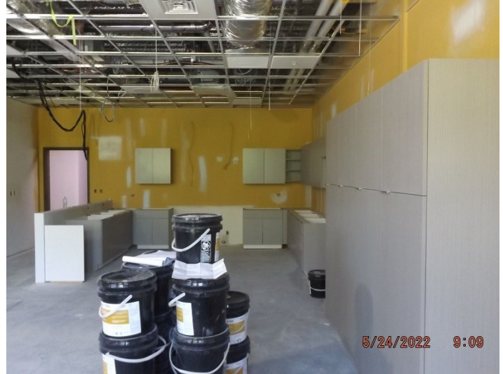
Photo depicts the progress of the Second floor kitchen.
