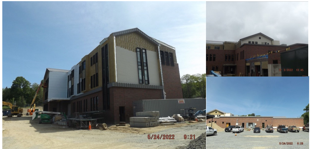
Pictures: Overall Site Progress
