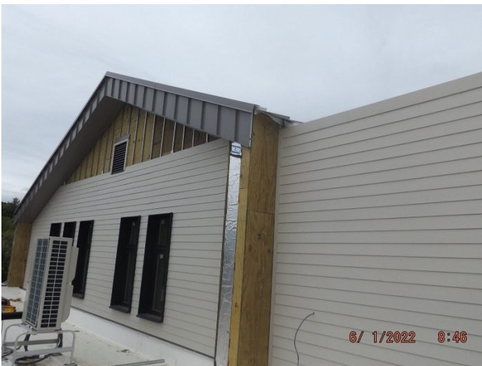
Photo depicts progress of the hardi plank siding
