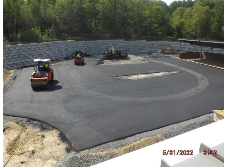
Photo depicts the installation of binder.
