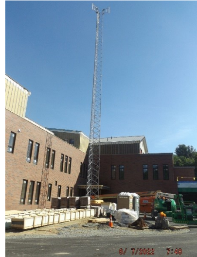
Photo depicts the installation of the communications tower.
