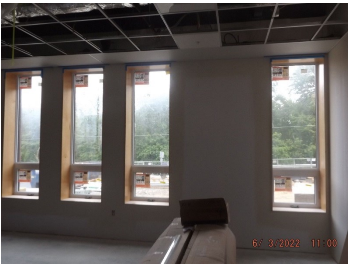
Photo depicts the progress of roll call.
