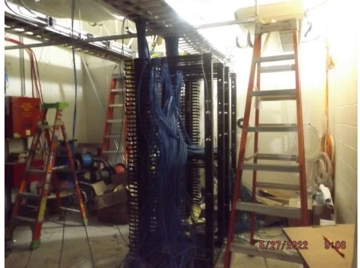
Photo depicts the progress of the server room.
