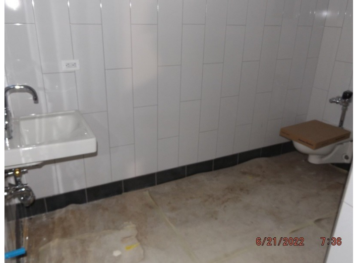
Photo depicts the progress of finish plumbing install.
