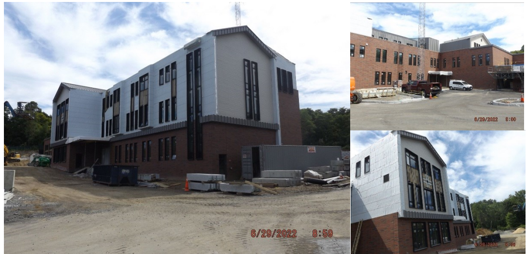
Pictures: Overall Site Progress
