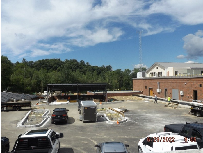
Photo depicts the progress of granite curb installation.
