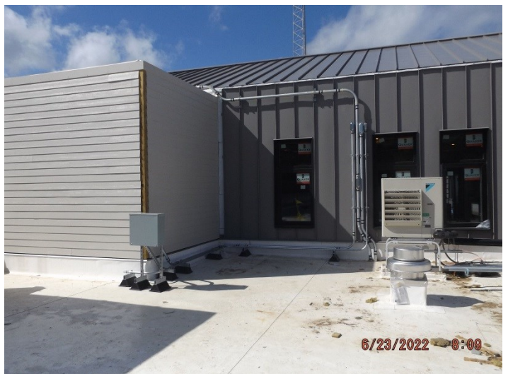
Photo depicts the installation of the solar infrastructure.
