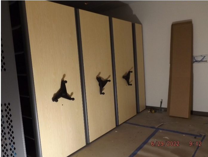
Photo depicts the progress of the mobile storage installation.
