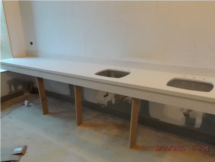
Photo depicts the progress of countertop installation.
