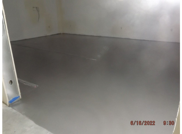
Photo depicts the progress of installation of epoxy flooring.
