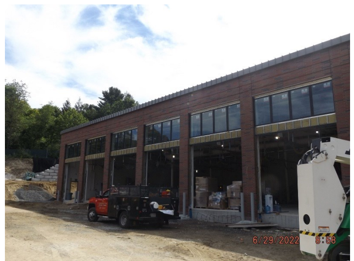
Photo depicts the progress of the exterior of the apparatus bay.
