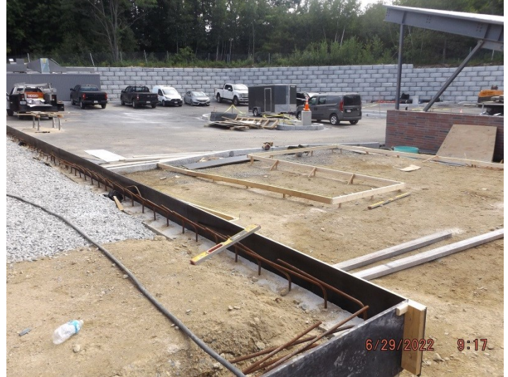
Photo depicts the preparation for concrete sidewalks.
