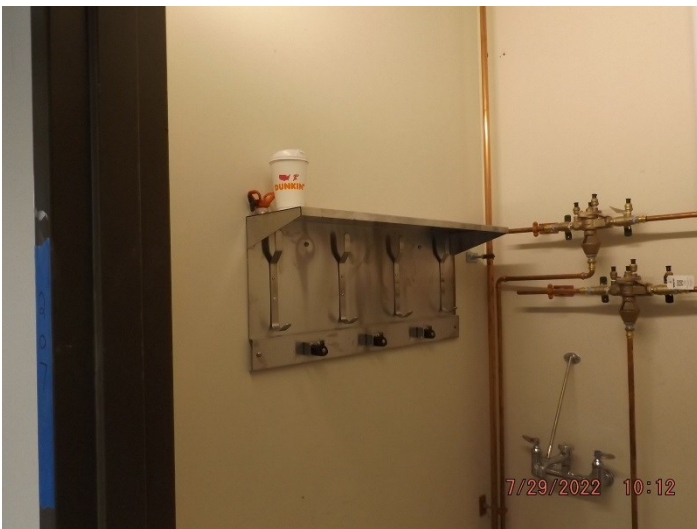
Photo depicts progress of the miscellaneous fixture installation.
