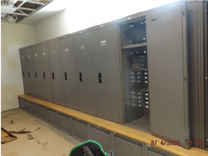
Photo depicts the progress of countertop installation.
