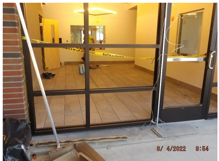
Photo depicts the progress of the lobby floor tiling.
