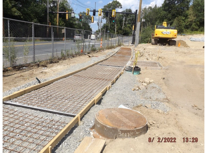
Photo depicts the preparation for the new sidewalk out front.
