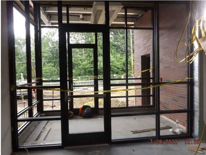
Photo depicts the progress of storefront vestibule installation.
