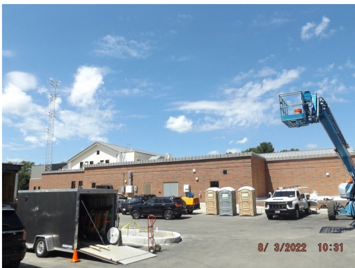
Photo depicts the progress of the exterior at the rear of the fire department side.
