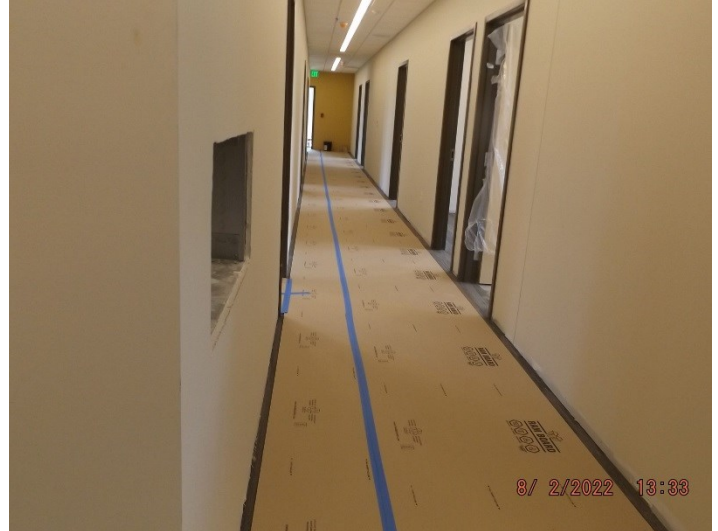
Photo depicts the third floor finished ceiling, walls and hallway flooring.
