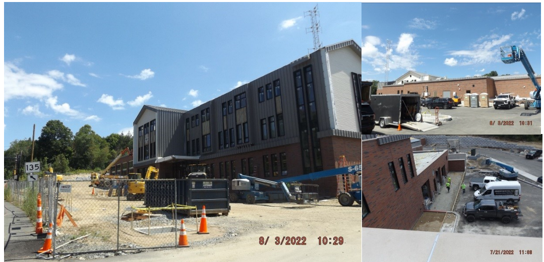
Pictures: Overall Site Progress
