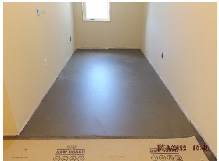
Photo depicts the installation of second floor resilient flooring.
