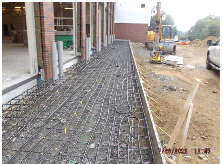
Photo depicts the preparation for the concrete apron at dispatch.
