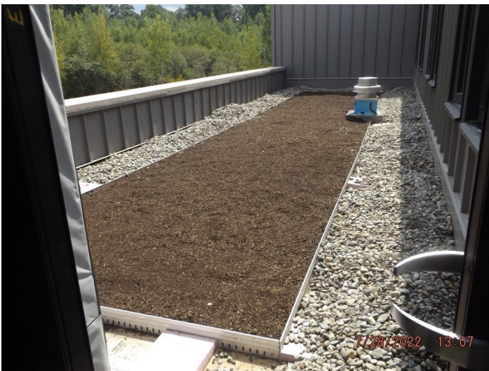
Photo depicts the progress of the upper green roof.
