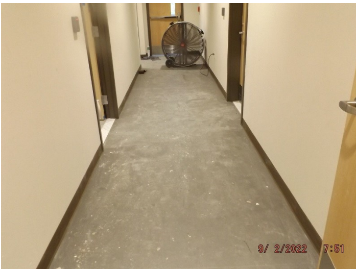
Photo depicts the progress of second floor on PD side
