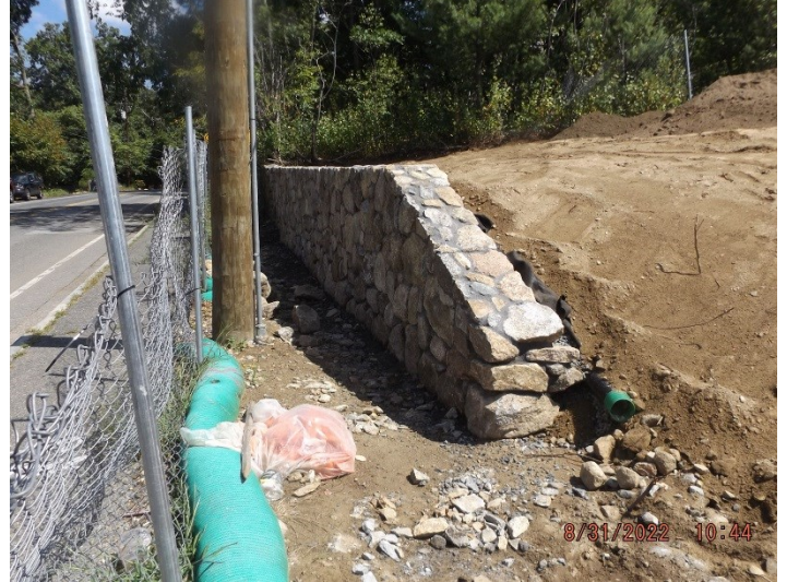
Photo depicts the completion of the new rock wall.
