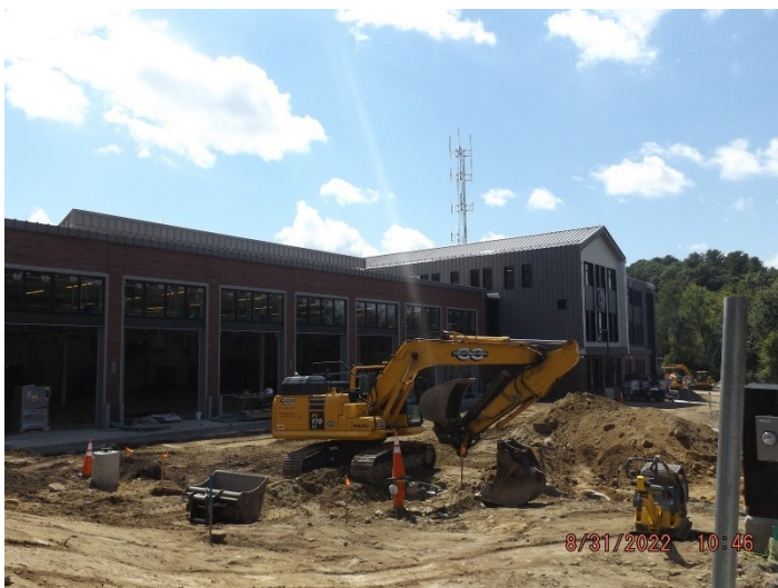
Photo depicts the progress of the front of the apparatus bay.
