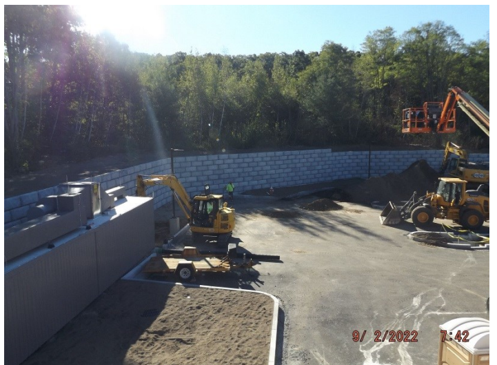
Photo depicts the progress of the loaming around the site.
