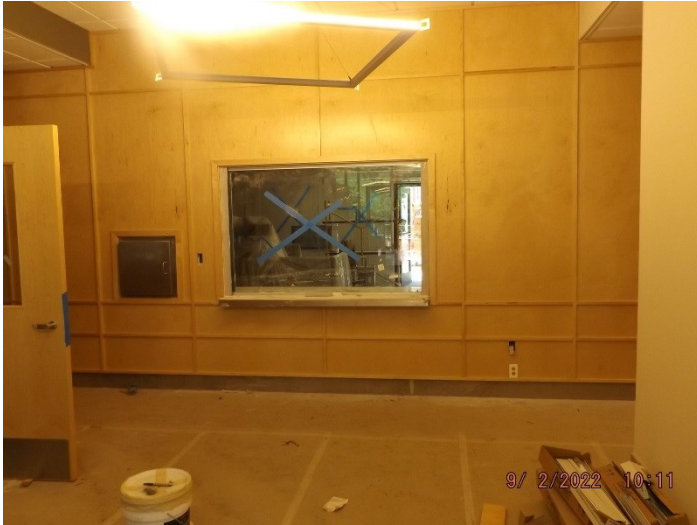
Photo depicts the progress of the lobby millwork
