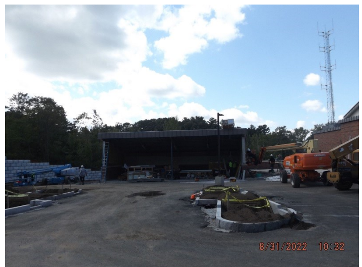
Photo depicts the progress of the car port.
