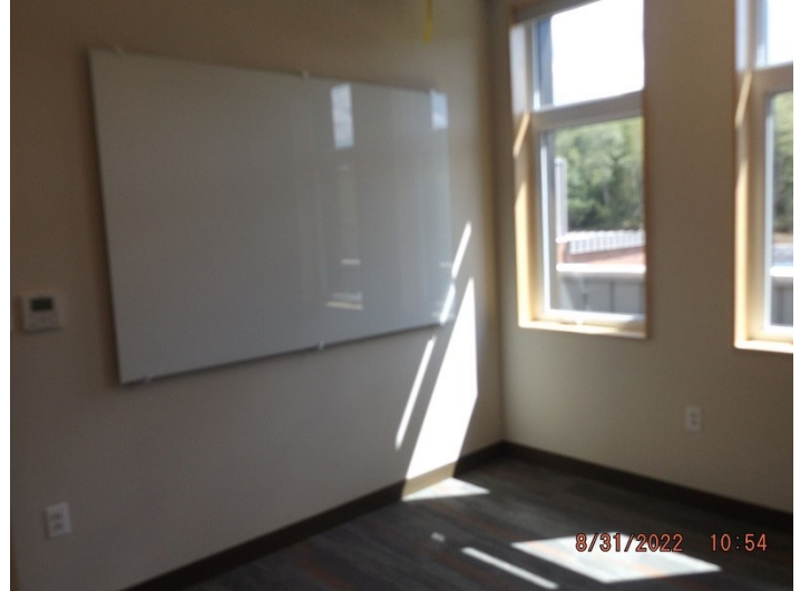
Photo depicts a completed third floor office on the PD side
