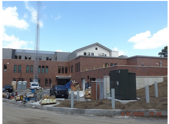
Photo depicts the progress the rear of the admin side of the building.
