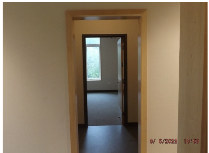
Photo depicts a completed second floor dorm room on FD side.
