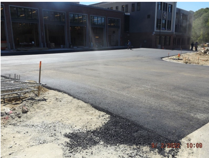
Photo depicts the progress of the paving.
