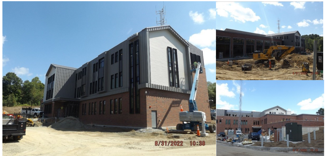
Pictures: Overall Site Progress
