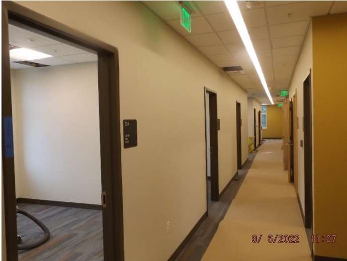
Photo depicts the progress of The third floor FD side
