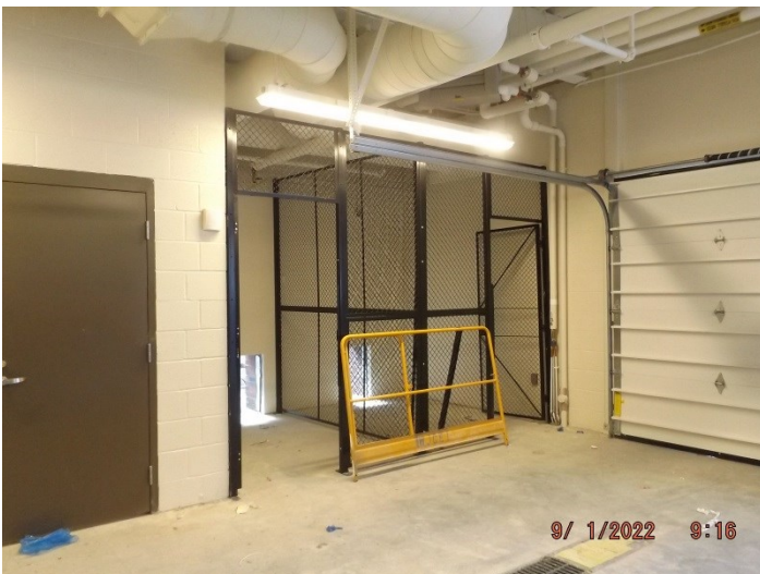
Photo depicts progress of the sally port area
