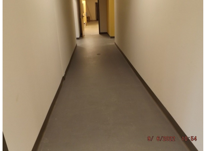
Photo depicts the progress of the first floor.
