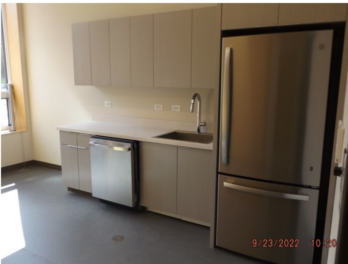
Photo depicts progress of the appliances
