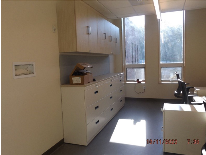
Photo depicts the progress of the furniture installation
