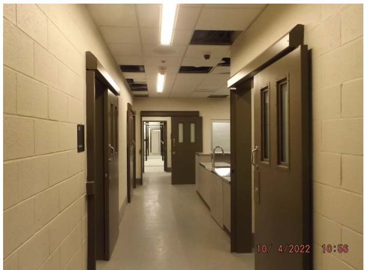
Photo depicts the substantially complete detention area.
