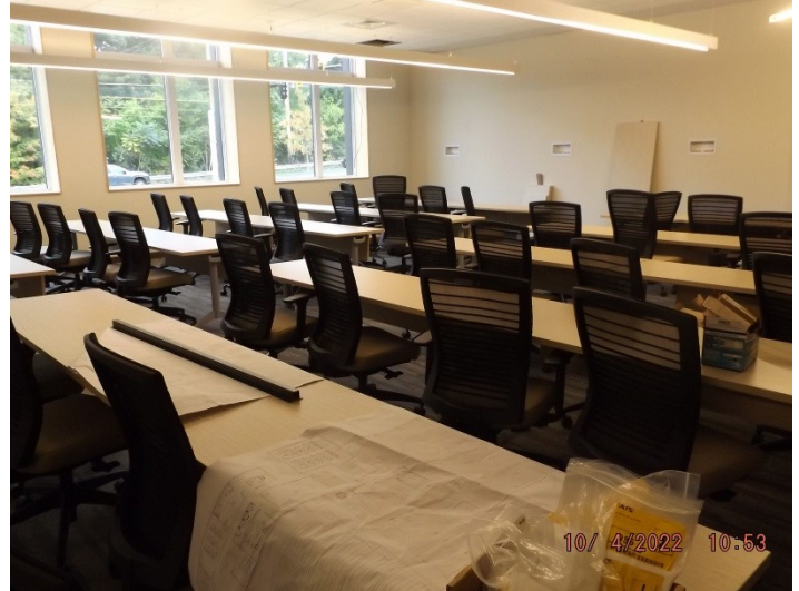
Photo depicts the progress of furniture install.
