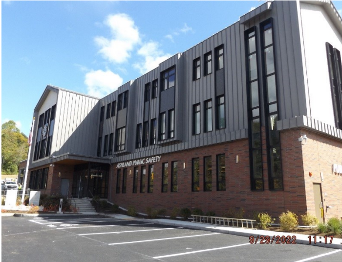
Photo depicts the substantially complete exterior.
