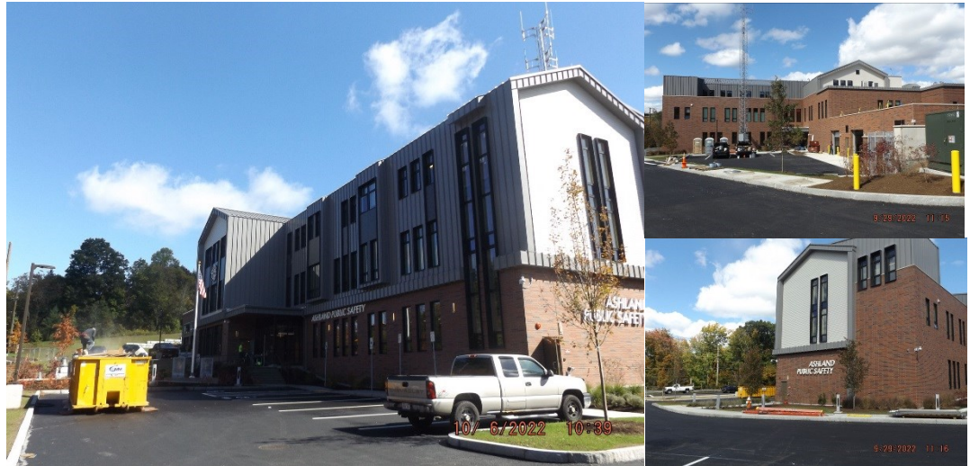
Pictures: Overall Site Progress
