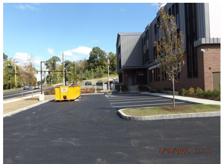
Photo depicts substantially complete exterior.
