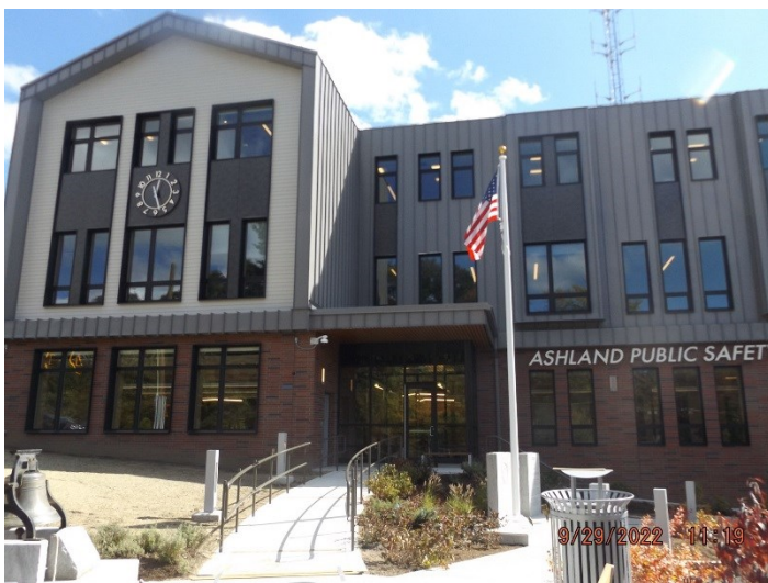
Photo depicts the substantially complete exterior.
