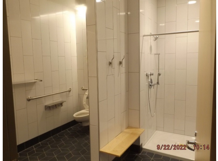
Photo depicts the substantially complete FD bathroom/shower.
