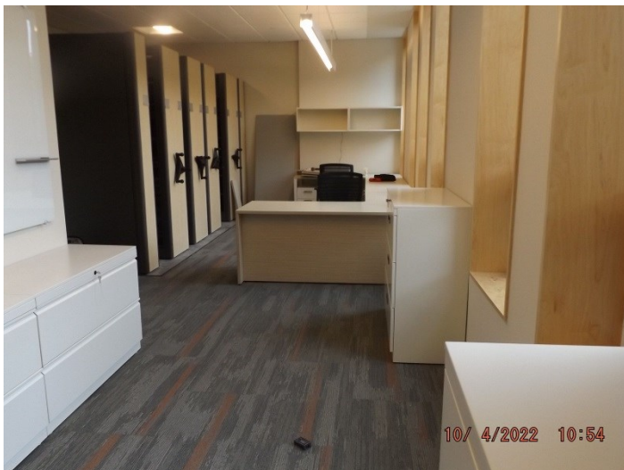
Photo depicts the progress of furniture installation.
