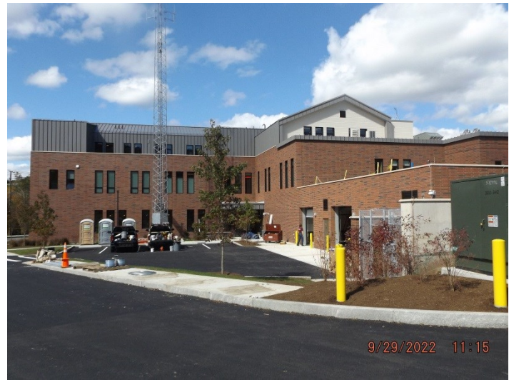
Photo depicts the substantially complete exterior.
