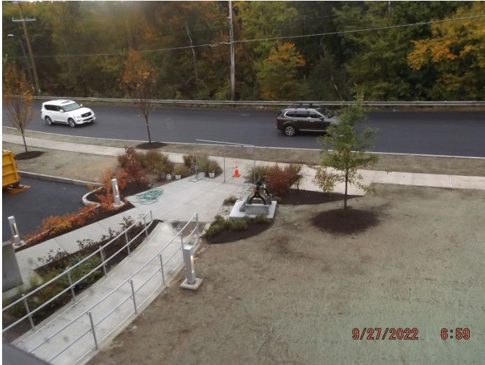
Photo depicts the substantially complete main entry and memorials.
