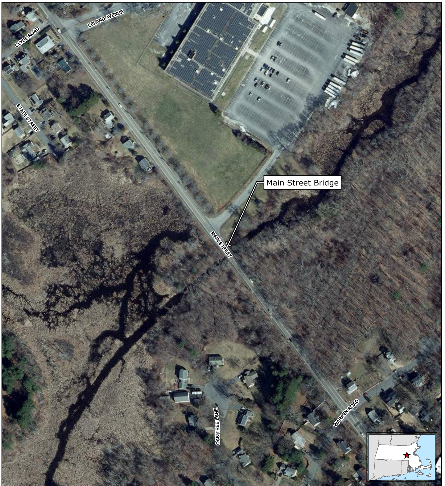
FIGURE 1 SITE AERIAL OVERVIEW
