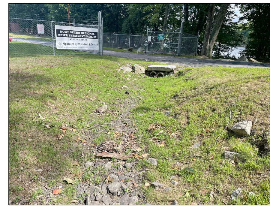
EXISTING GRASS & STONE SWALE NORTH OF DRIVEWAY
