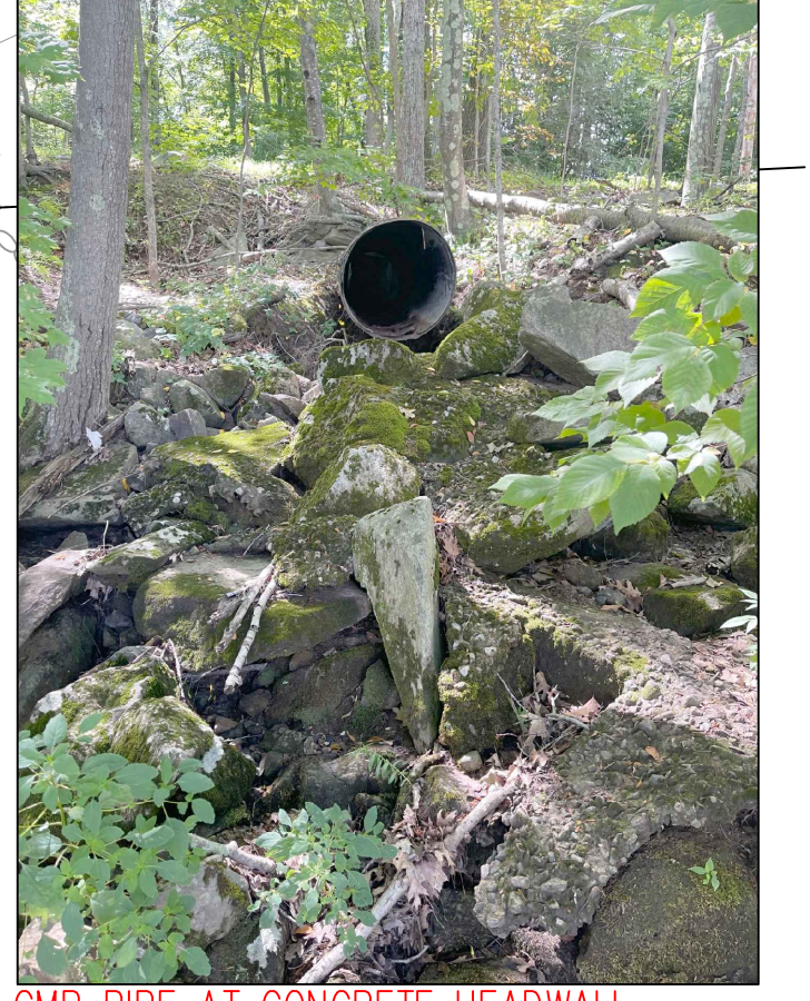
EXISTING CMP PIPE AT CONCRETE HEADWALL
