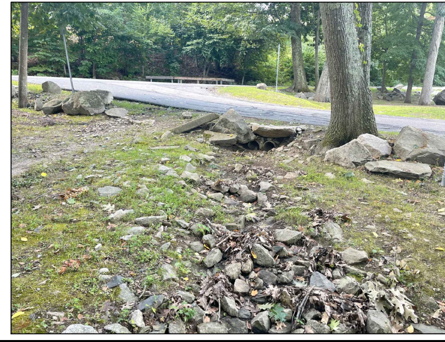
EXISTING GRASS & STONE SWALE NORTH OF DRIVEWAY
