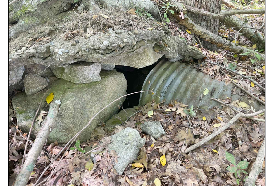
EXISTING CMP PIPE AT CONCRETE HEADWALL
