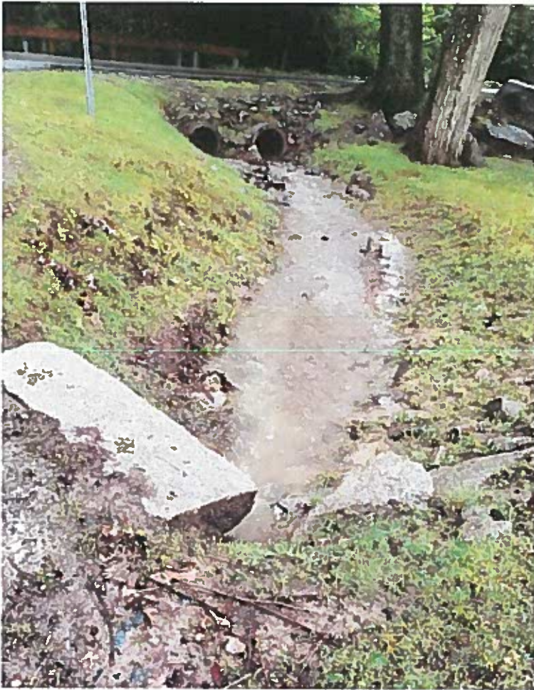
7/12/2021: turbidity water from culverts under Howe Street, leading to the culvert under the driveway at the Water Plant, Howe Street, Ashland, and then to the Hopkinton Reservoir.
