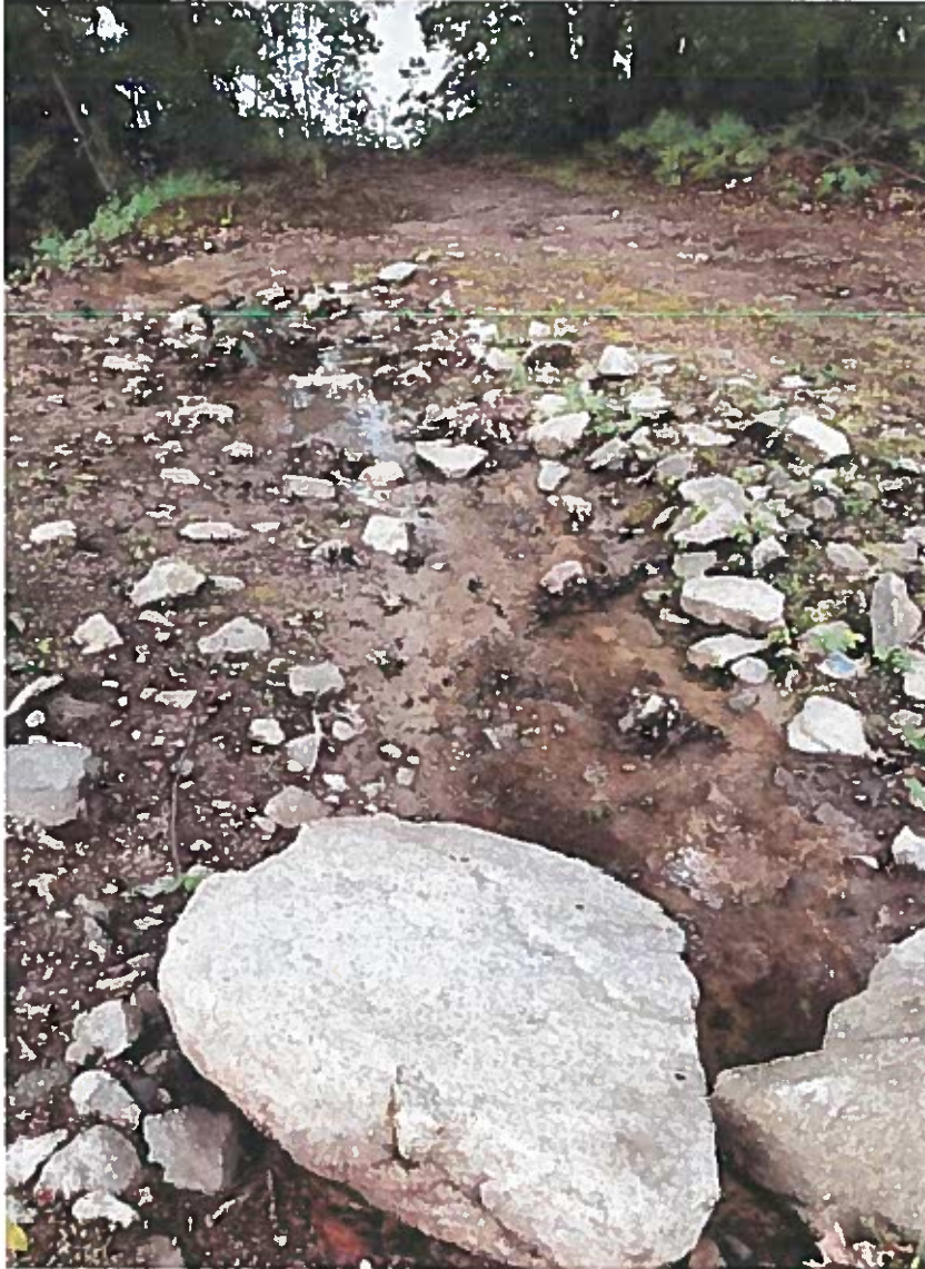
7/8/2021: Fine Sediment in Discharge. Taken at the water treatment plant, Ashland, facing the Hopkinton Reservoir.
