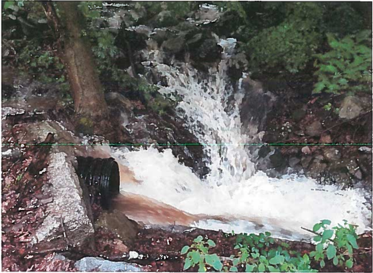
7/9/2021: Headwall to Howe Street culverts near the treatment plant.
