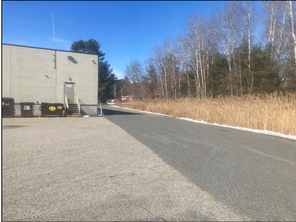
Photo E-1. A view facing northwest of the project site from behind the building at 200 Butterfield Lane. March 1, 2023.
