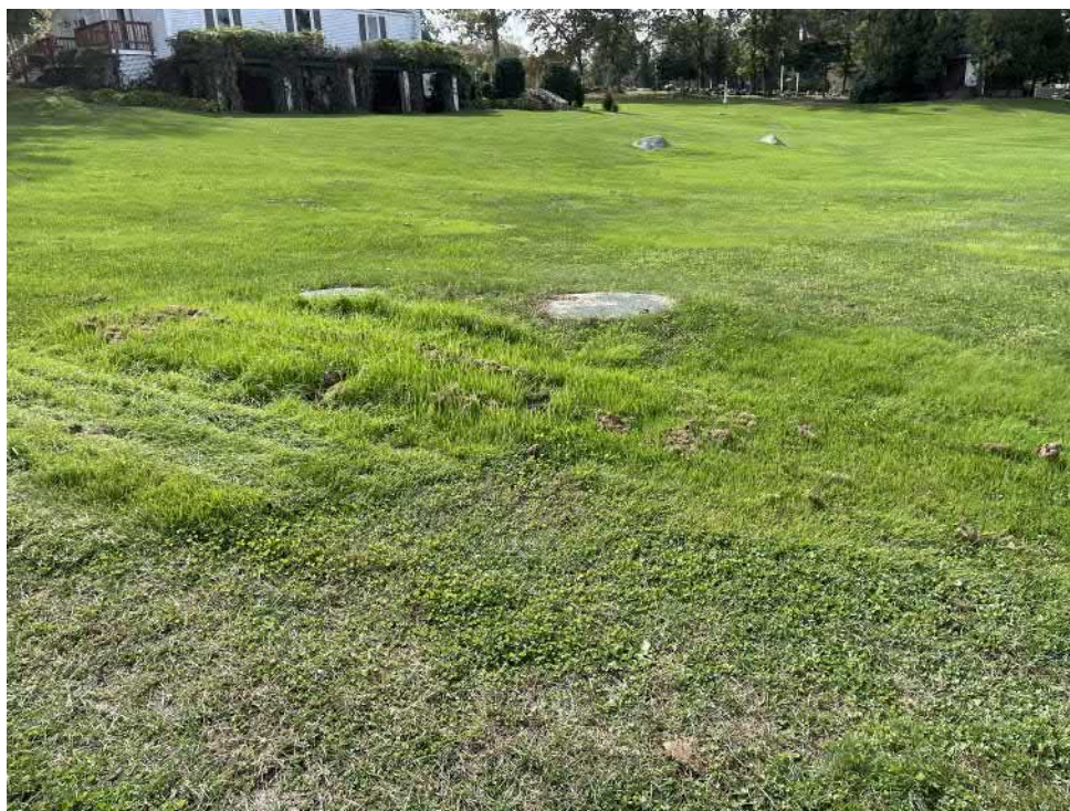
View of the Middle Pump Station—facing south.
