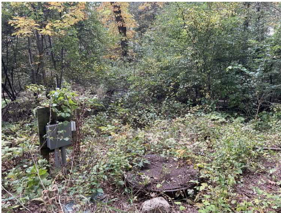
View of the Lower Pump Station—facing southwest.
