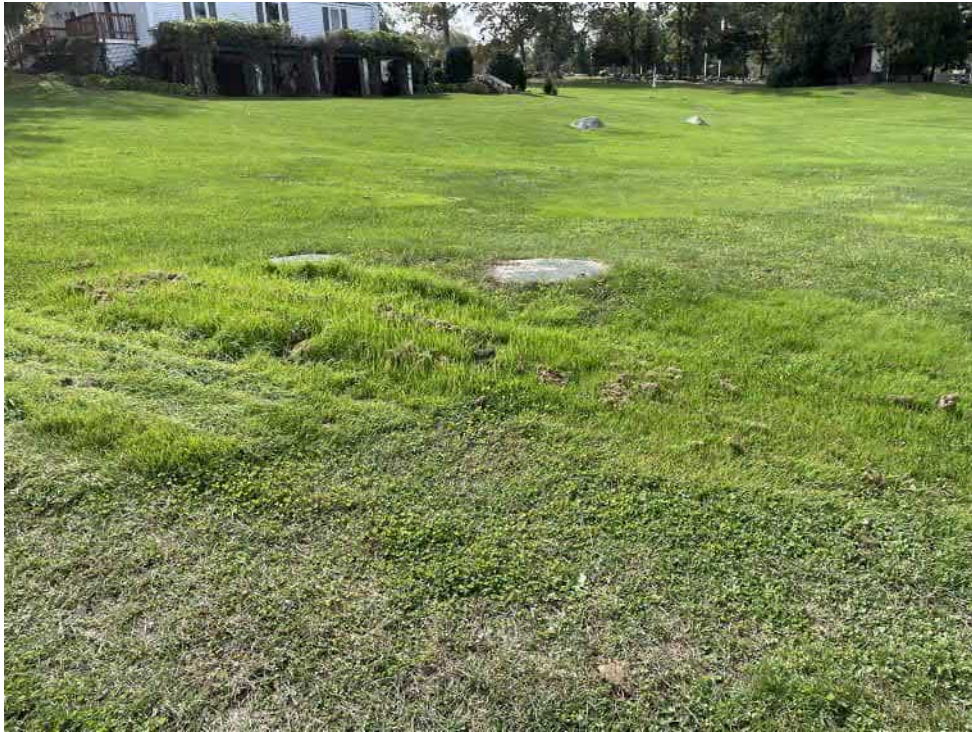
View of the Middle Pump Station—facing south.
