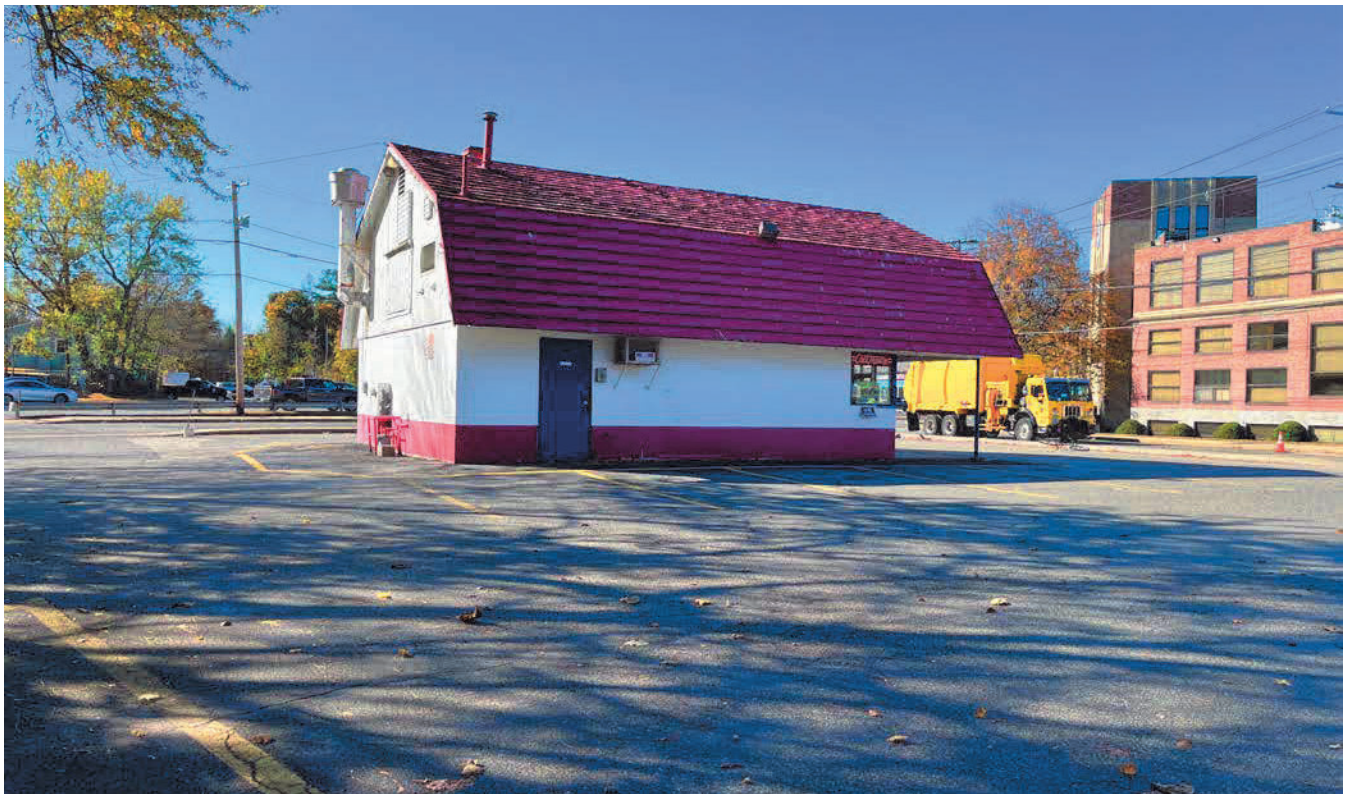
Photo #2: Photo looking at existing building with Chestnut Street at the left of the building and Union Street to the right..
