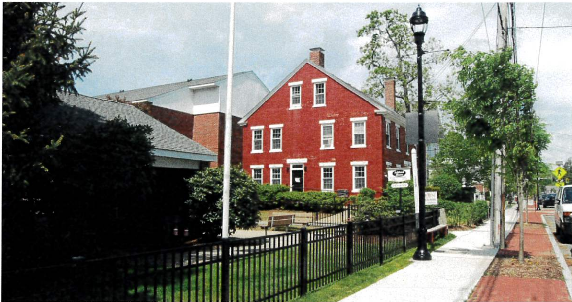
Photo 8. View looking northwest toward Rev. James McIntire House (119 Main St.) and attached Ashland House apartment building (senior housing).
