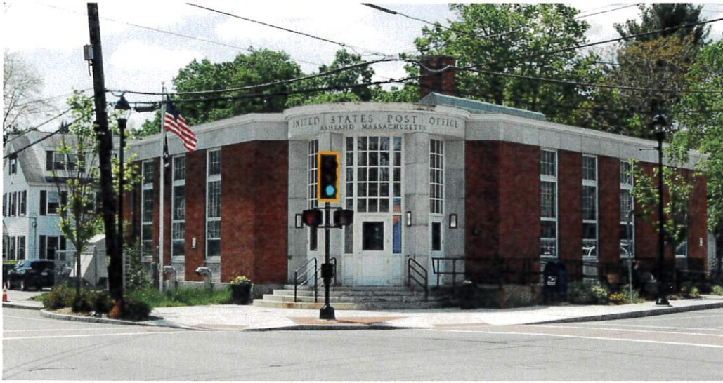
Photo 3. View looking south toward Ashland Post Office (205 Main St.).
