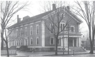
Ashland Town Hall – Main Street (1905)
