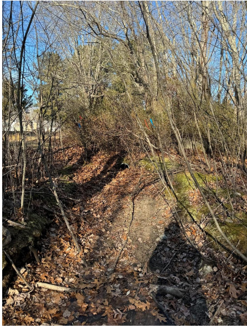
Photo 1 - 12" PVC Outlet Pipe from Northern Portion of BVW
