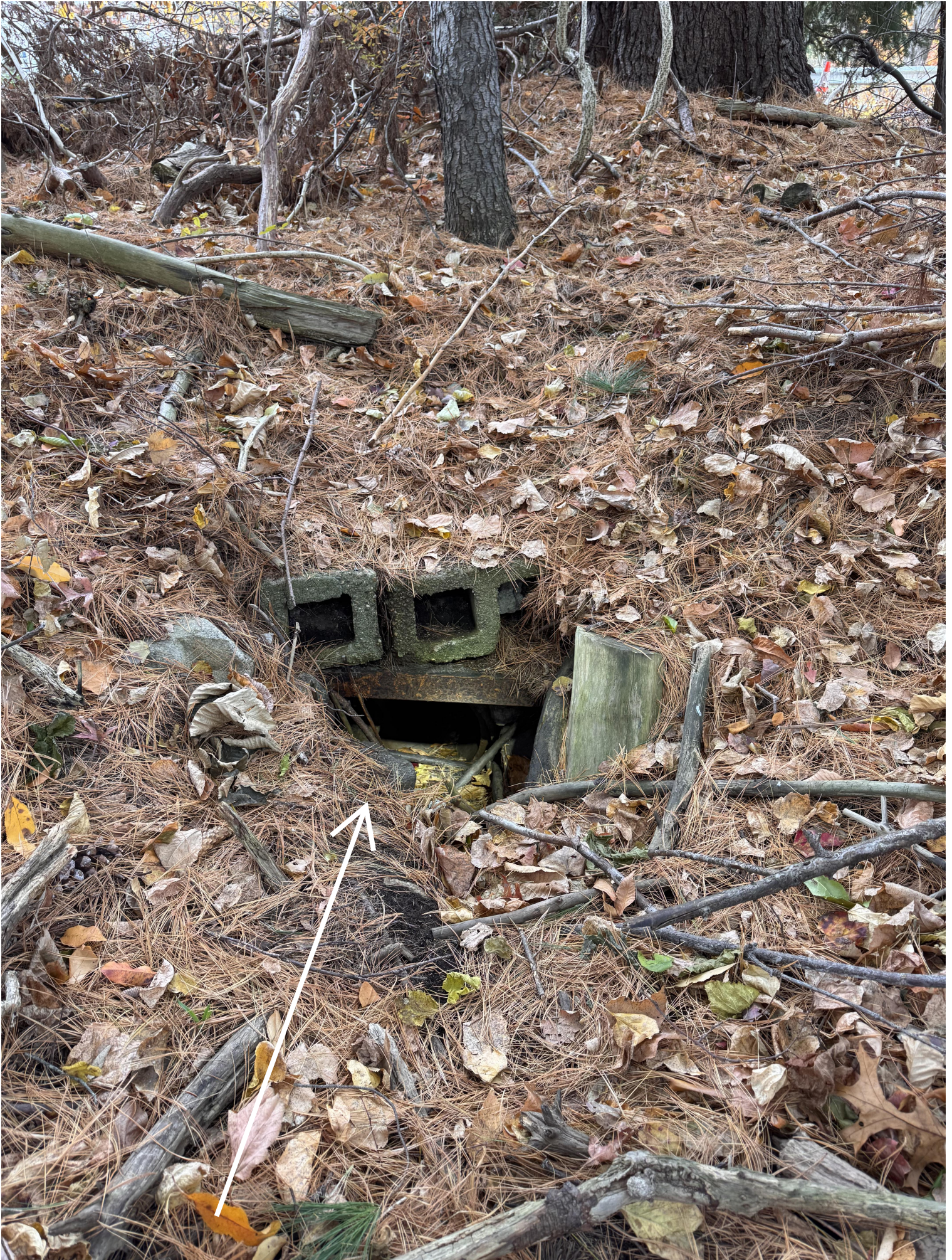
Inlet side of culvert
