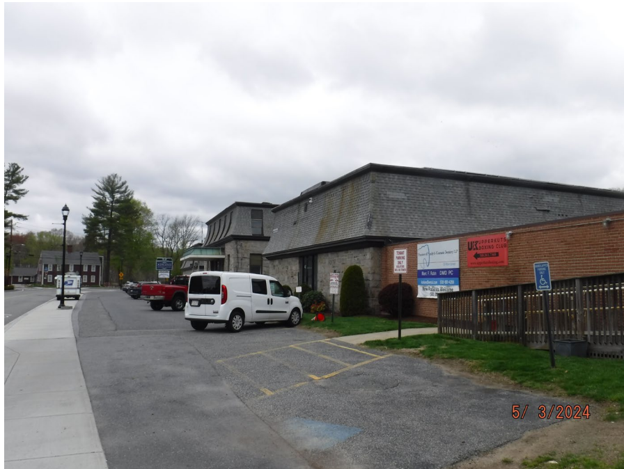
Photograph 25: View of existing degrading mill structures along Main Street, facing north.
