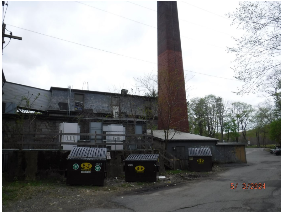
Photograph 17: Existing Chimney Stack to remain in proposed conditions, facing northwest.
