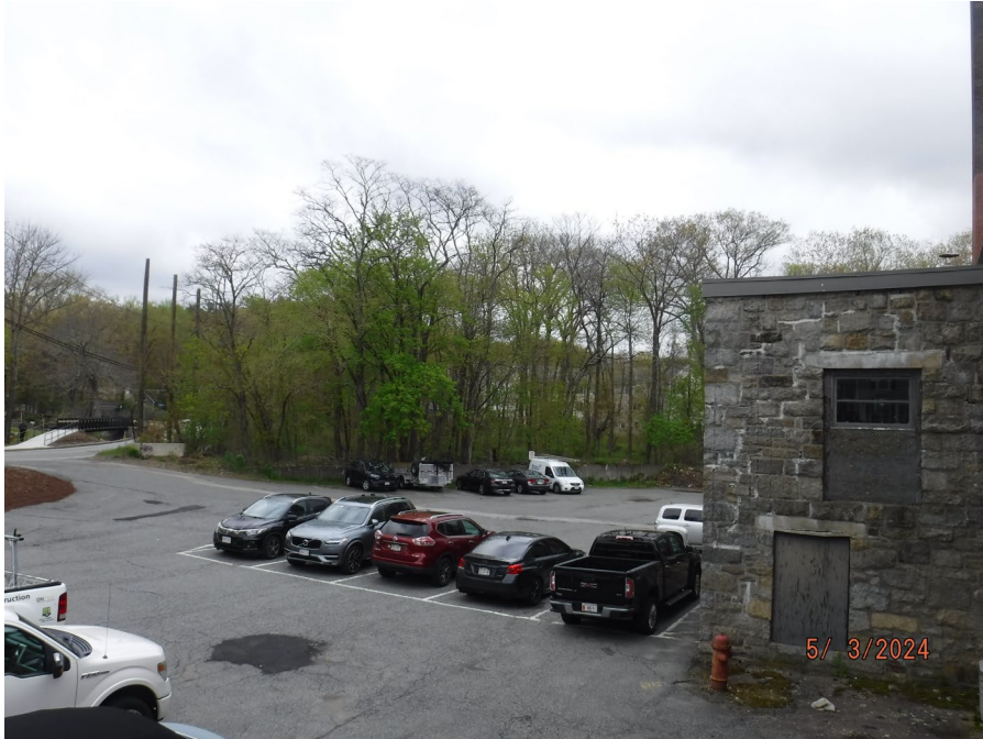
Photograph 23: View of impervious parking lot and existing mill structure, facing north.
