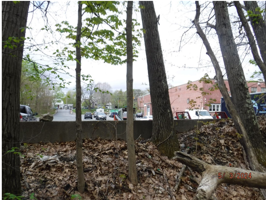
Photograph 9 : View of retaining wall, parking lot, and mill building, facing west towards Main Street approximately near flags MAHW#3 and #4.
