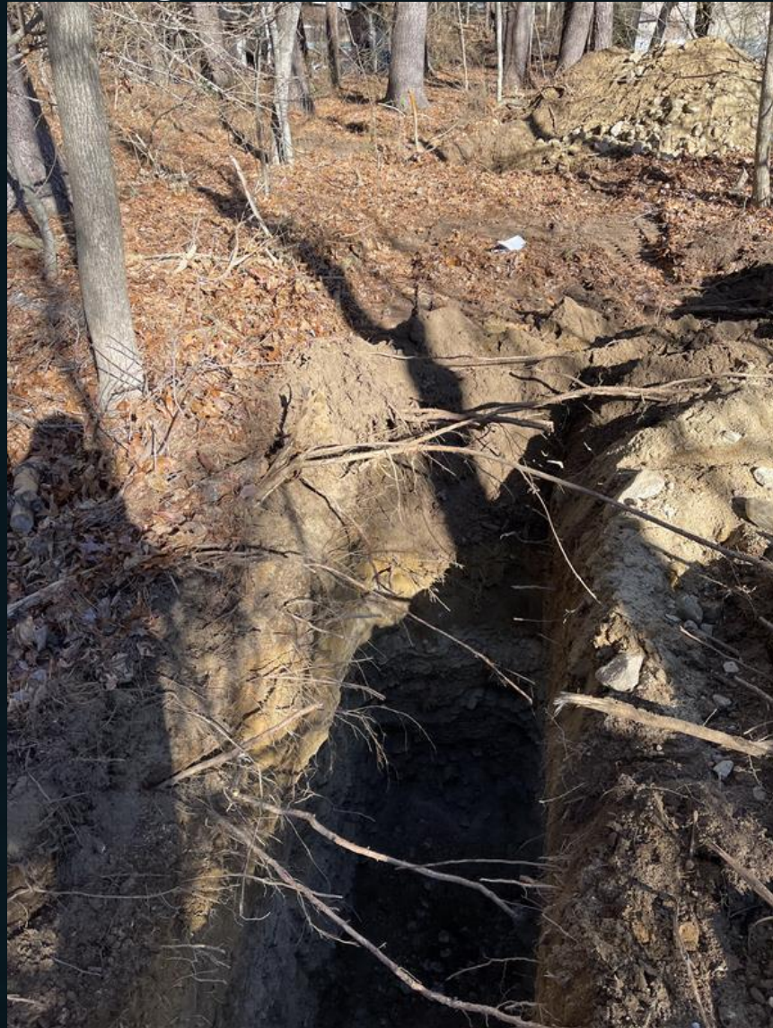
Image 6 – Behind 8 Ballard Rd Looking North
