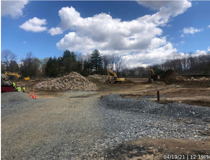
Photo depicts the progress of rock removal.
