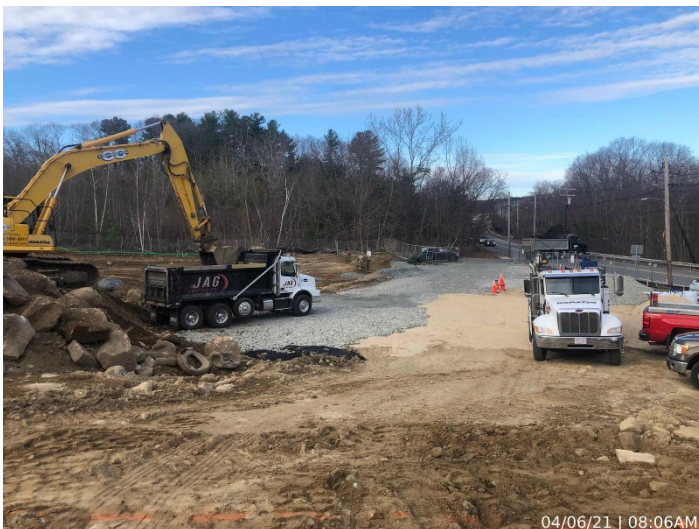
Photo depicts the crushed stone entry for trucking.
