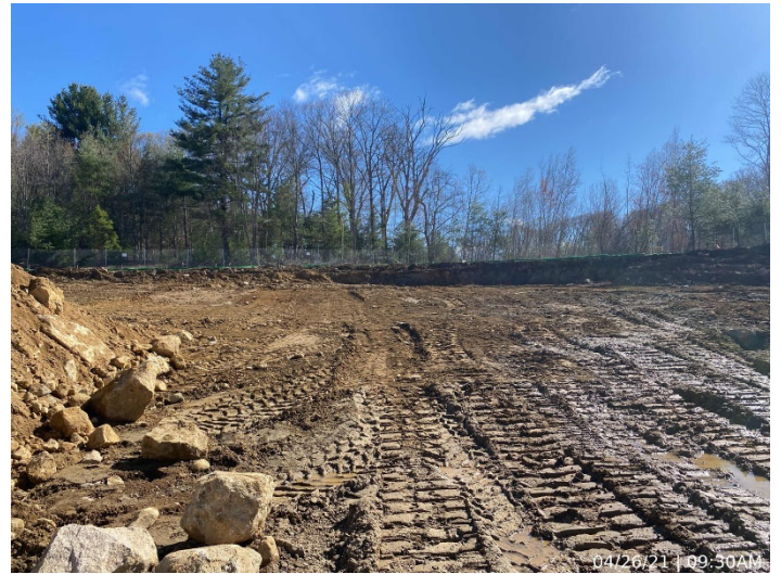
Photo depicts the progress at the rear of the Site
