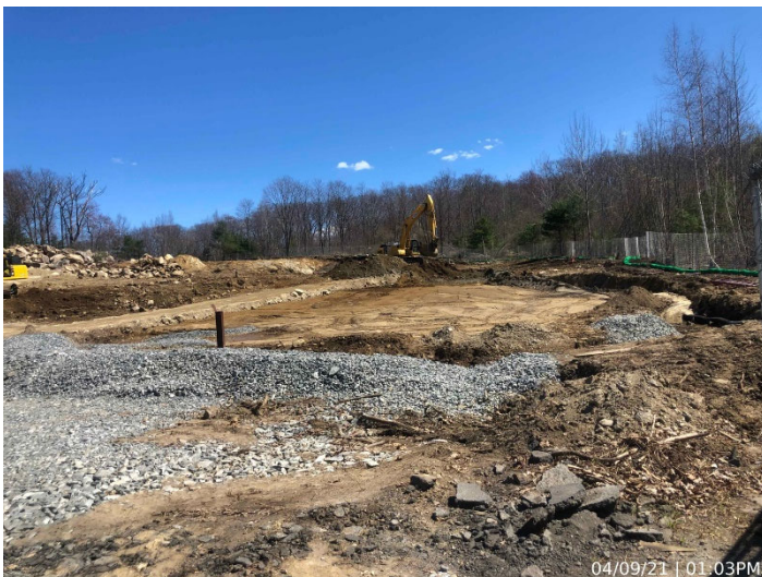
Photo depicts the progress of stock piling of loam
