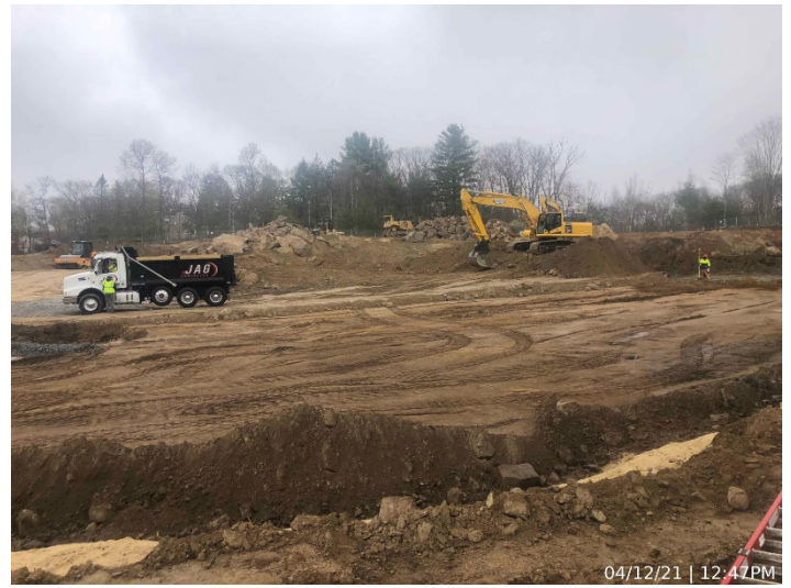
Photo depicts the overall progress of the site.
