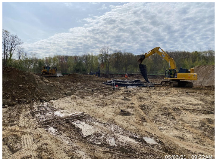
Photo depicts the laying of mats for test blast.
