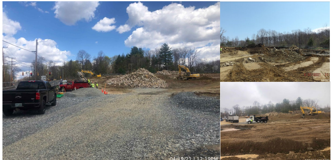
Pictures: Overall Site Progress
