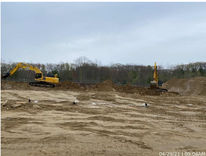
Photo depicts the progress of probing in preparation for blasting.
