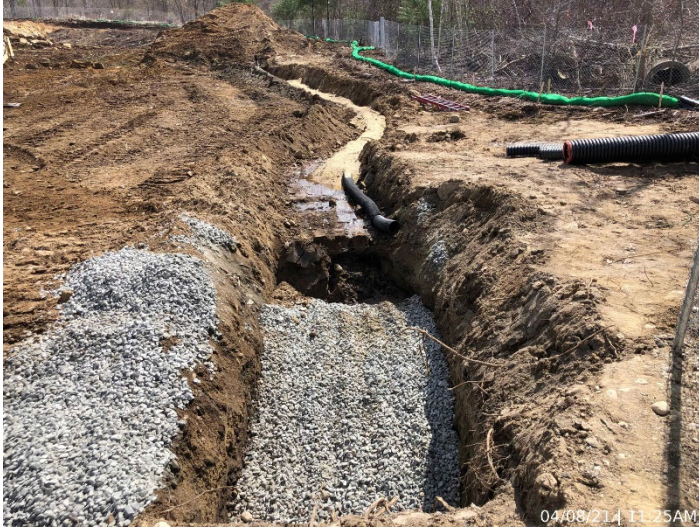
Photo depicts trenching to help direct groundwater.
