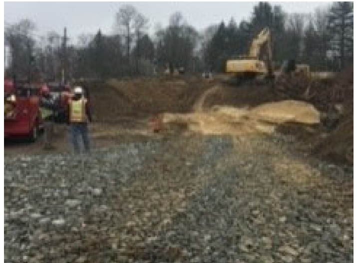
Photo depicts the progress of the Site
