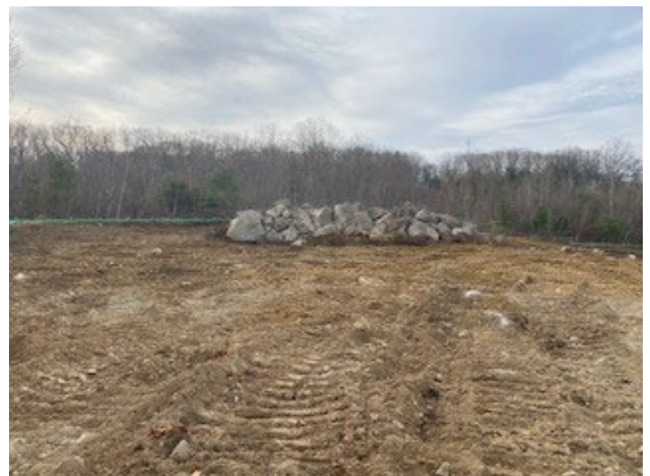
Photo depicts the progress of the Site
