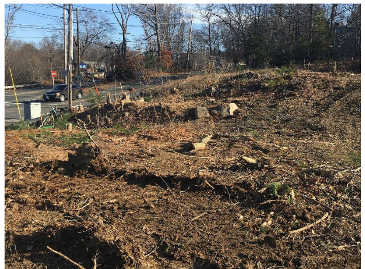
Photo depicts progress of the site.
