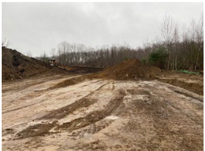
Photo depicts the progress of the Site
