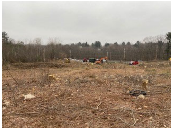
Photo depicts the progress of the Site
