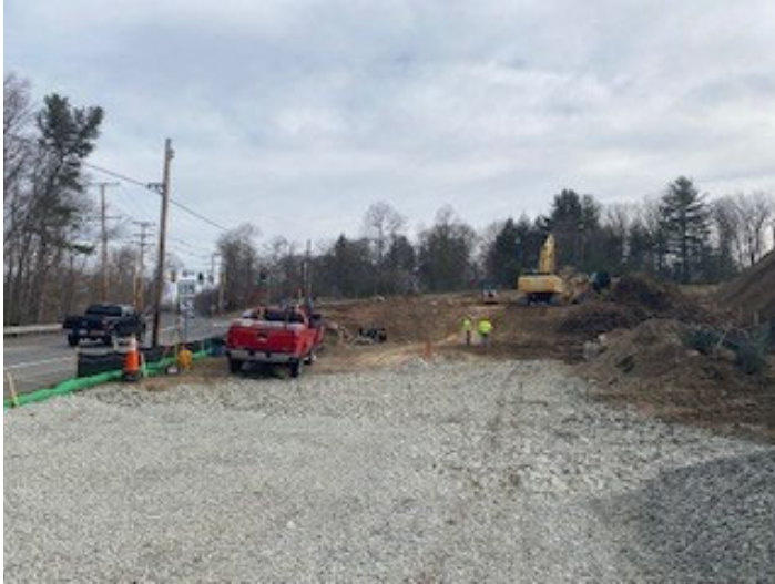
Photo depicts the progress of the Site
