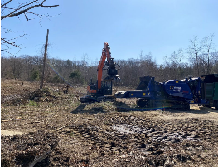
Photo depicts the progress of the Site
