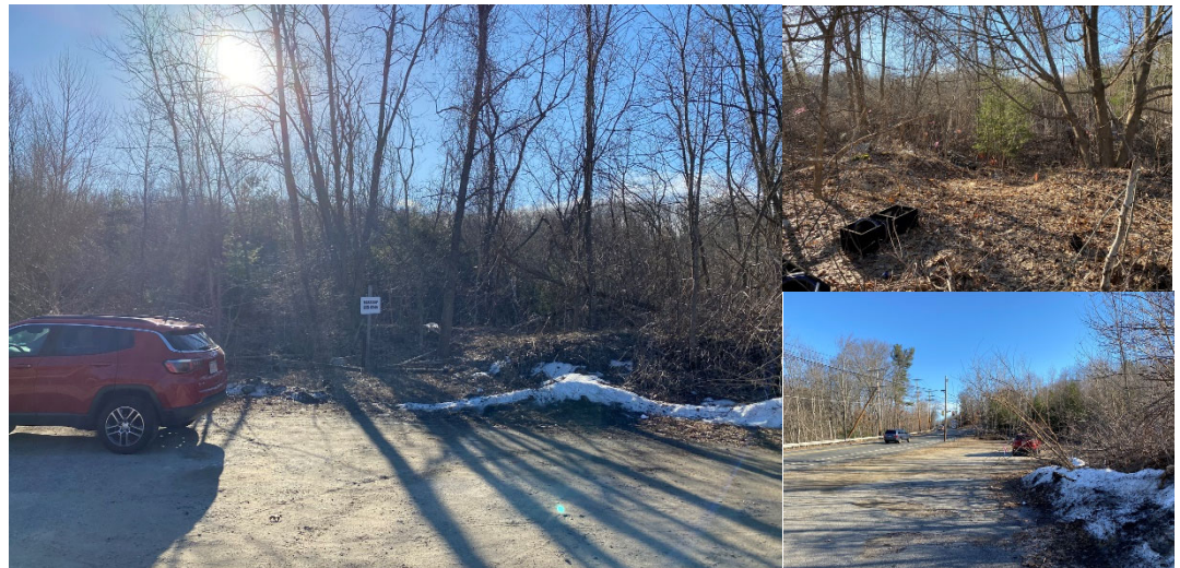
Pictures: Overall Site Progress
