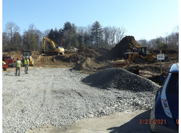
Photo depicts the progress of the Site
