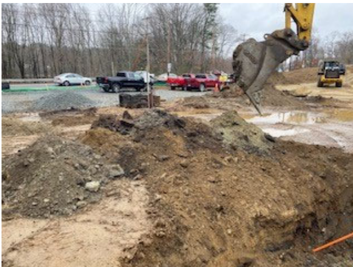
Photo depicts the progress of the Site
