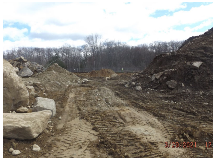
Photo depicts the progress of exterior.
