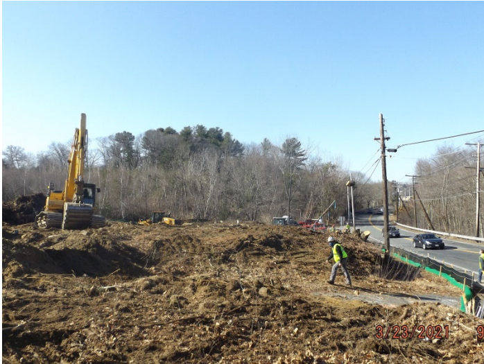
Photo depicts the progress of the Site
