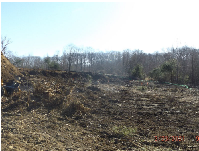
Photo depicts the progress of the Site
