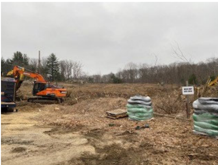
Photo depicts the progress of the site.
