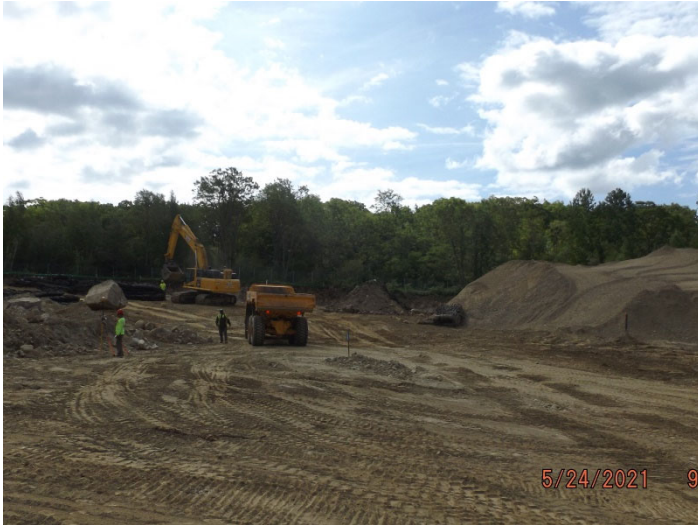
Photo depicts the progress of rock crushing, and stockpiling
