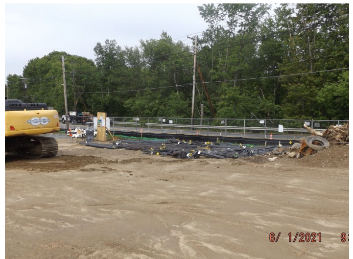
Photo depicts the delivery of rebar for concrete footings.
