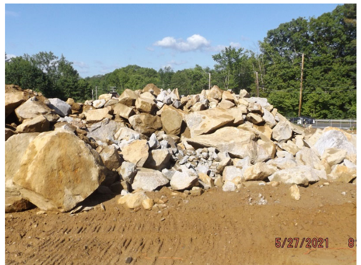
Photo depicts the progress of stockpiling of ledge.
