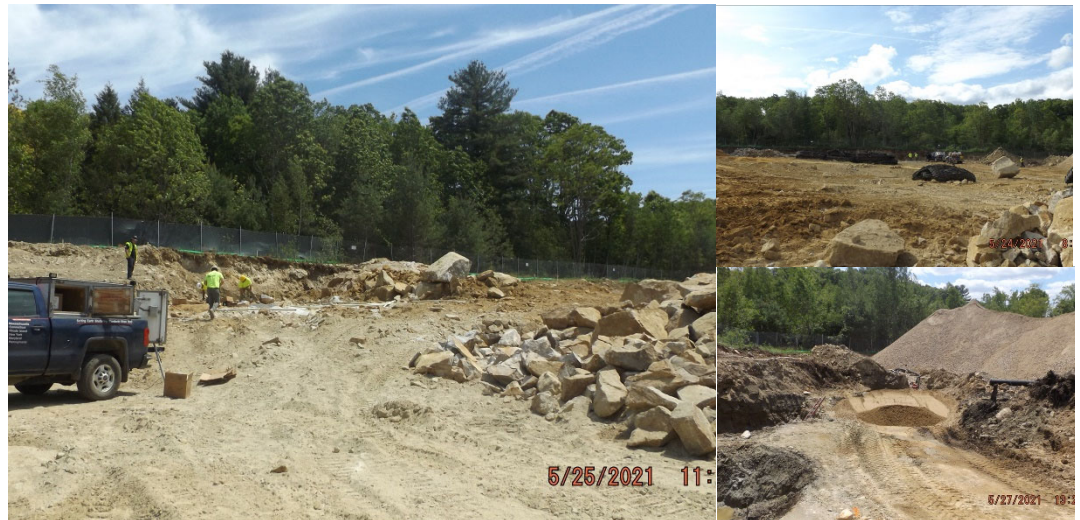
Pictures: Overall Site Progress
