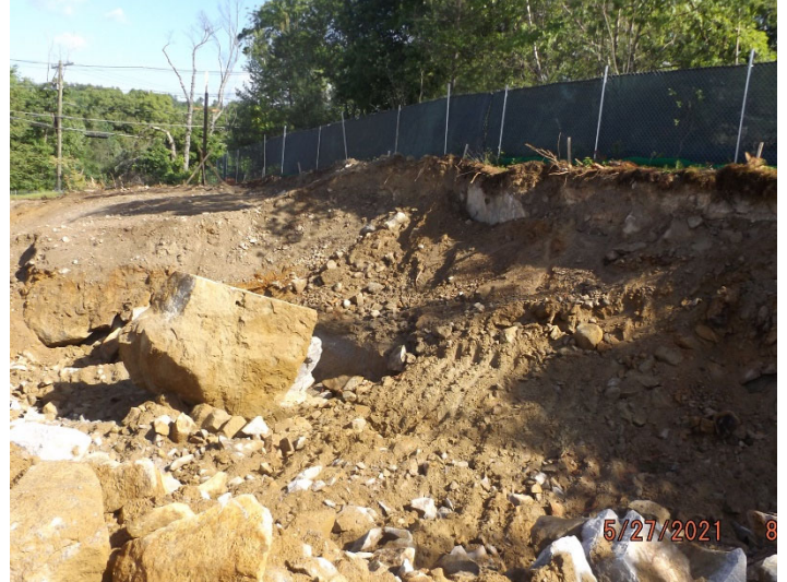
Photo depicts the dislodged ledge after blasting.
