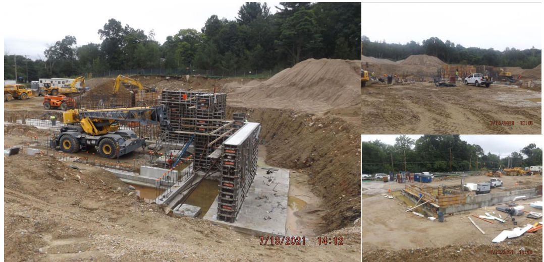
Pictures: Overall Site Progress
