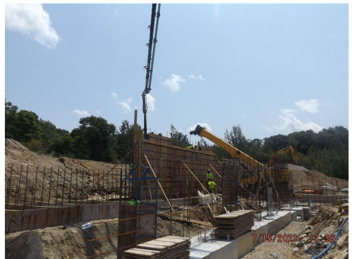
Photo depicts the concrete pour for the high foundation walls.
