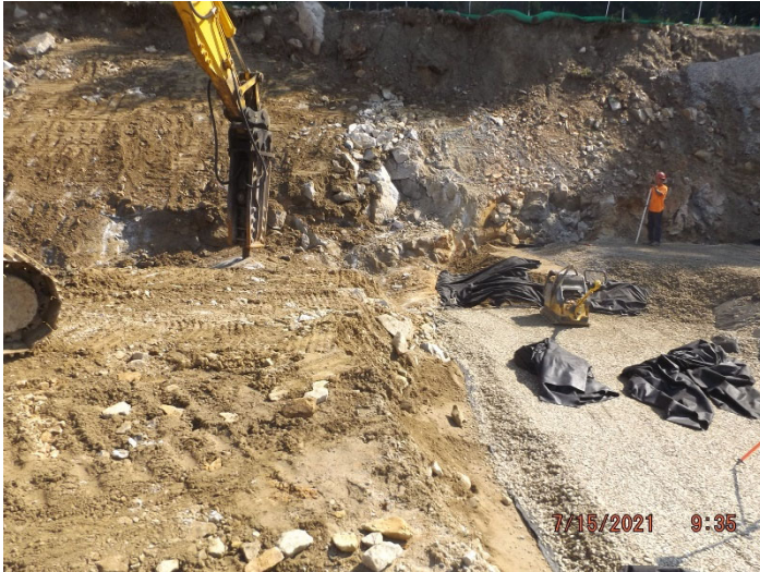
Photo depicts the under footing preparations
