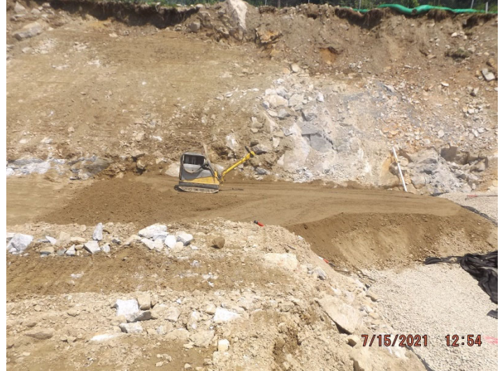
Photo depicts the under footing preparations.
