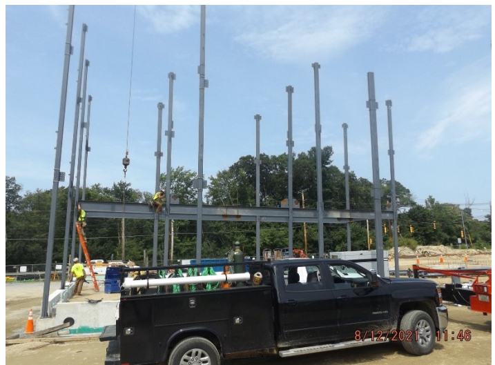
Photo depicts the steel erection.
