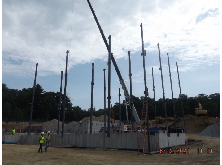
Photo depicts the steel erection.
