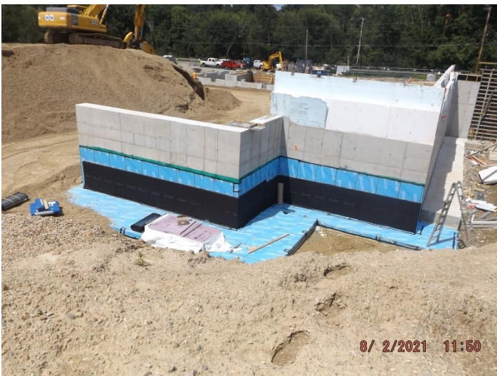
Photo depicts the progress of waterproofing.
