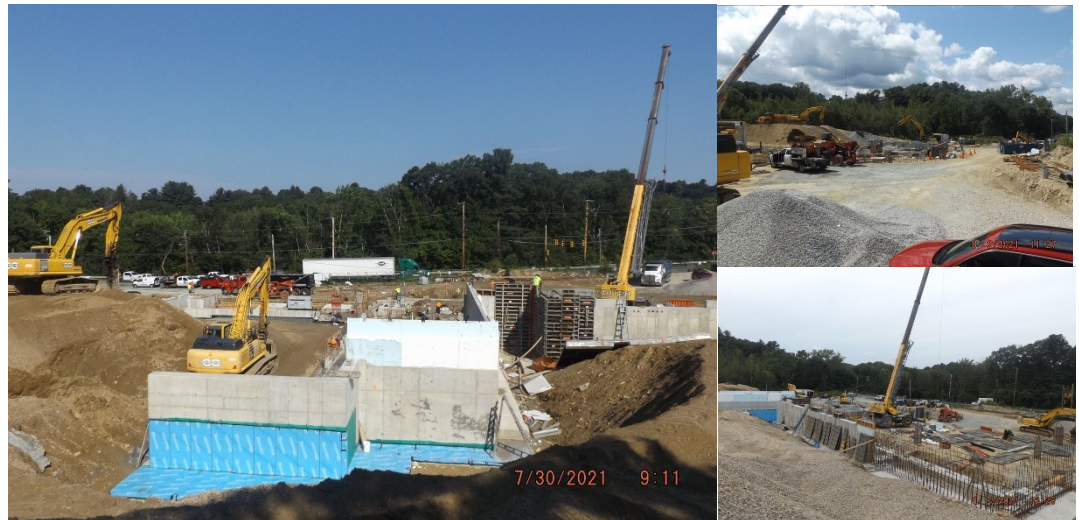
Pictures: Overall Site Progress
