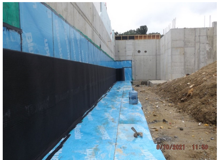
Photo depicts the progress of waterproofing.
