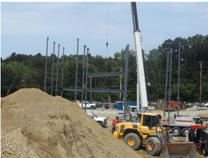
Photo depicts the steel erection.
