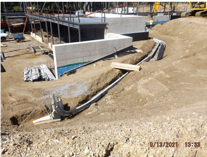
Photo depicts the progress of primary electrical conduits.
