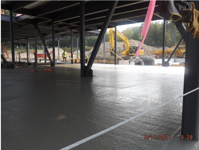
Photo depicts the second floor slab pour.
