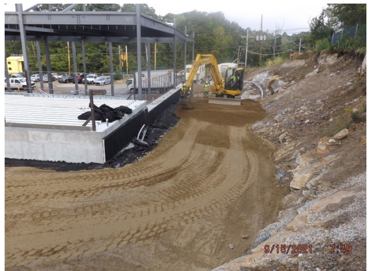
Photo depicts the site progress.
