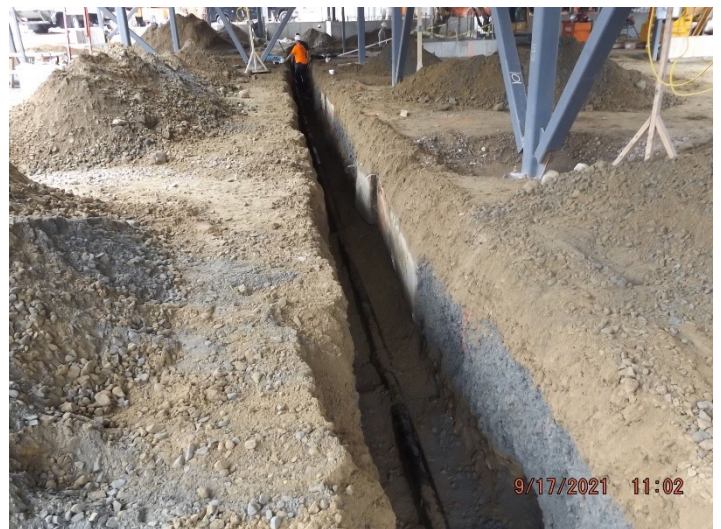
Photo depicts the progress of under ground plumbing.
