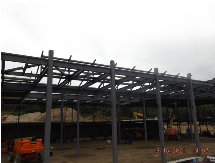
Photo depicts the progress of steel on the apparatus bay side.
