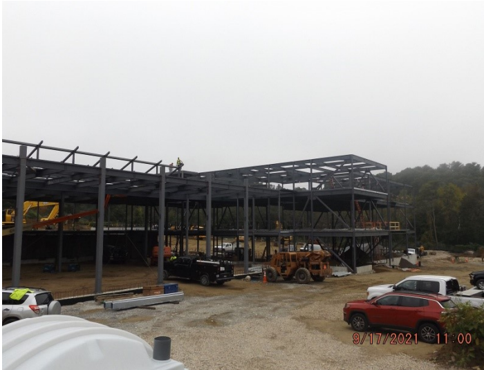
Photo depicts the progress of steel overall.
