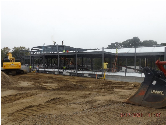
Photo depicts site progress.
