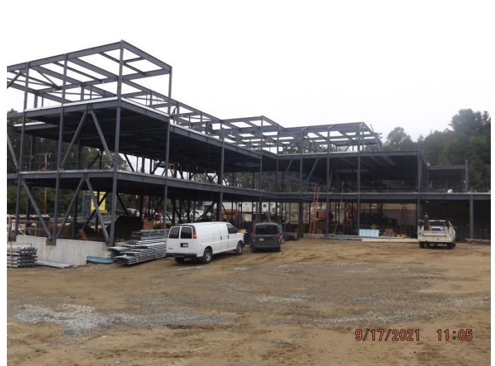
Photo depicts the progress of steel on the admin. side.
