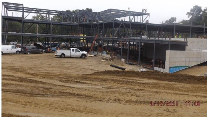
Photo depicts the site progress
