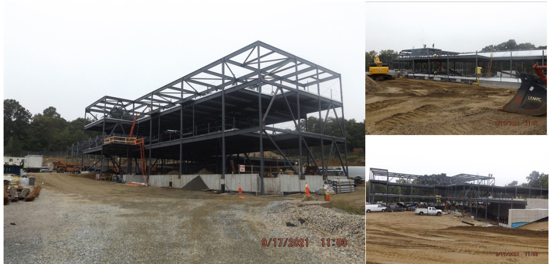
Pictures: Overall Site Progress
