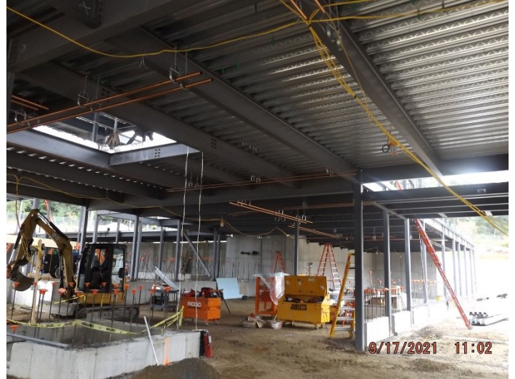
Photo depicts the progress of HVAC piping.
