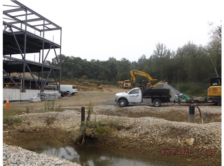
Photo depicts the site progress.
