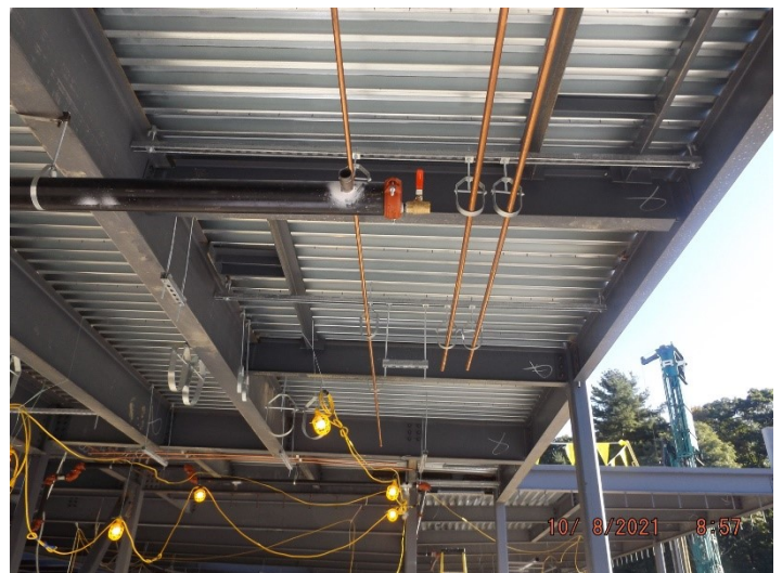
Photo depicts the progress rough electrical, fire protection and HVAC.
