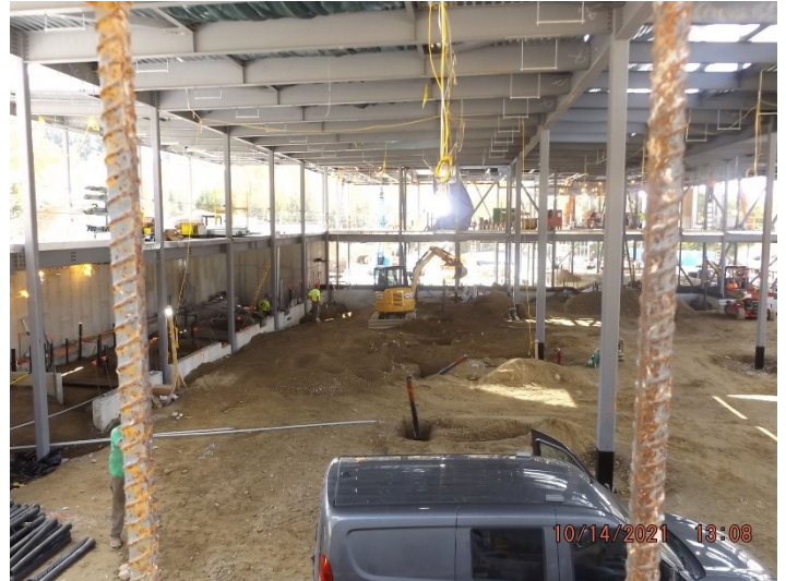
Photo depicts the overall apparatus bay progress.
