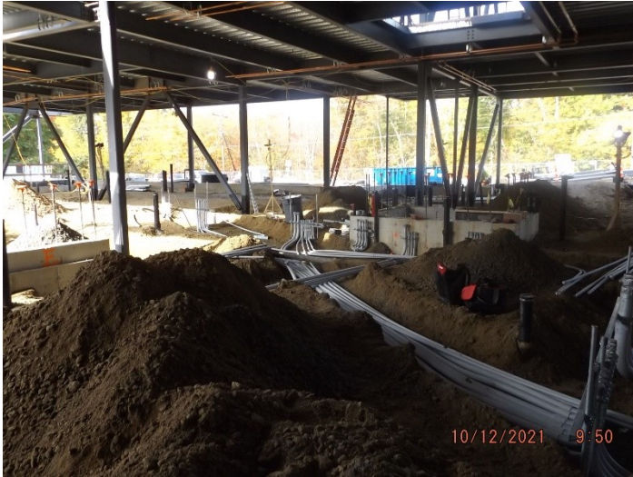
Photo depicts the under slab electrical progress.
