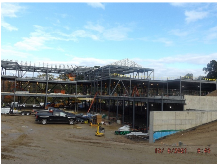
Photo depicts the progress of steel and framing.
