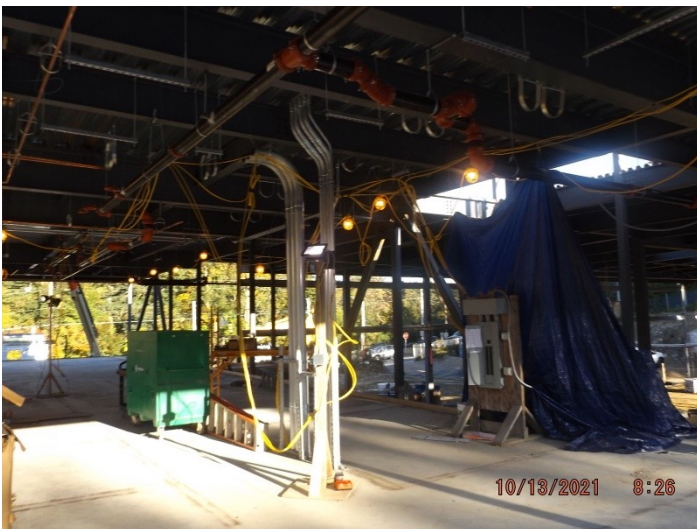
Photo depicts the progress rough electrical, fire protection and HVAC on second floor.
