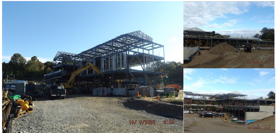
Pictures: Overall Site Progress
