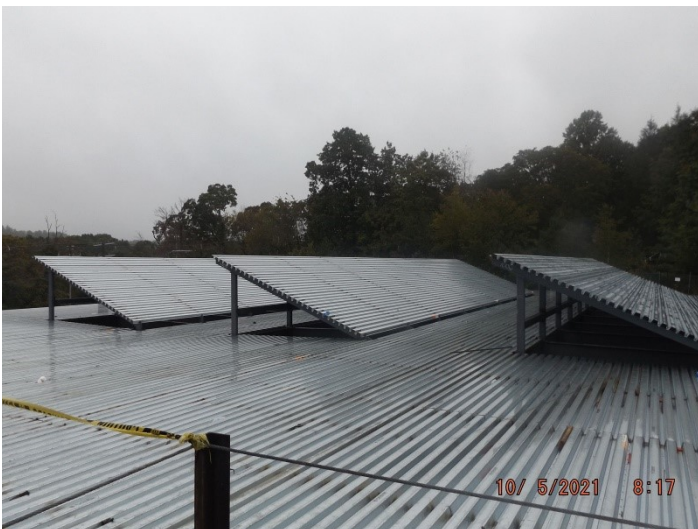
Photo depicts progress of the roof decking.
