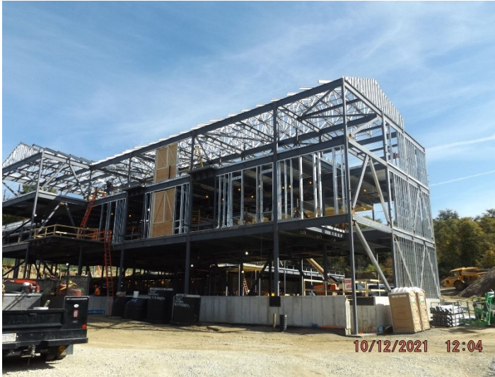
Photo depicts the progress of steel and framing.
