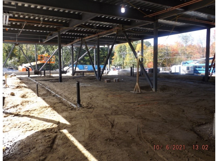
Photo depicts the progress of under slab plumbing and back filling.
