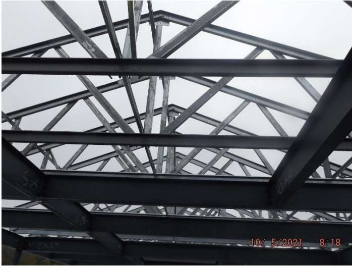
Photo depicts the progress of the trusses
