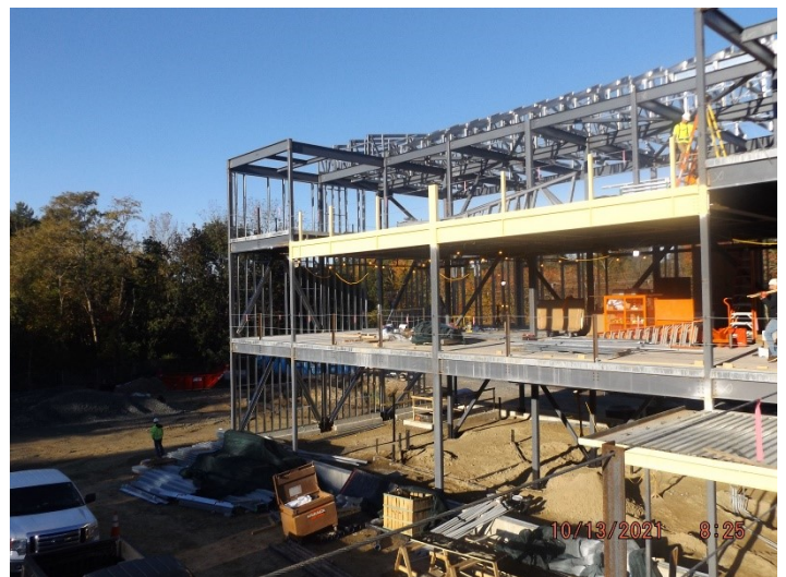
Photo depicts the progress of the insulative coating
