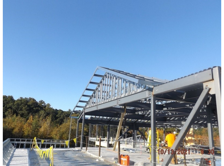
Photo depicts the progress of the trusses.
