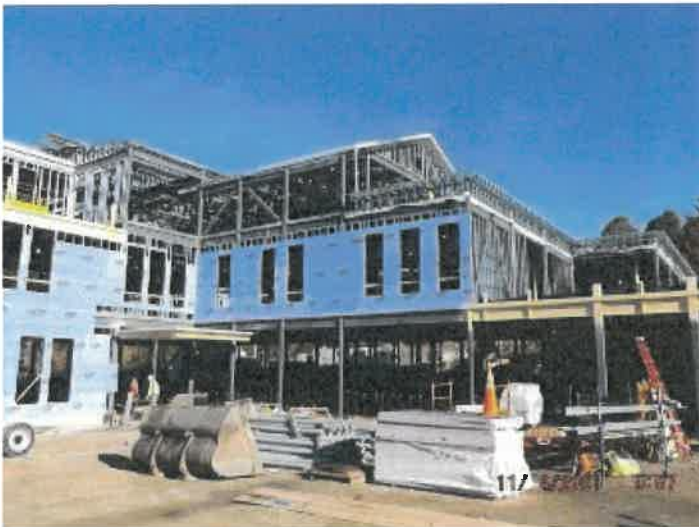
Photo depicts the progress of exterior sheathing.
