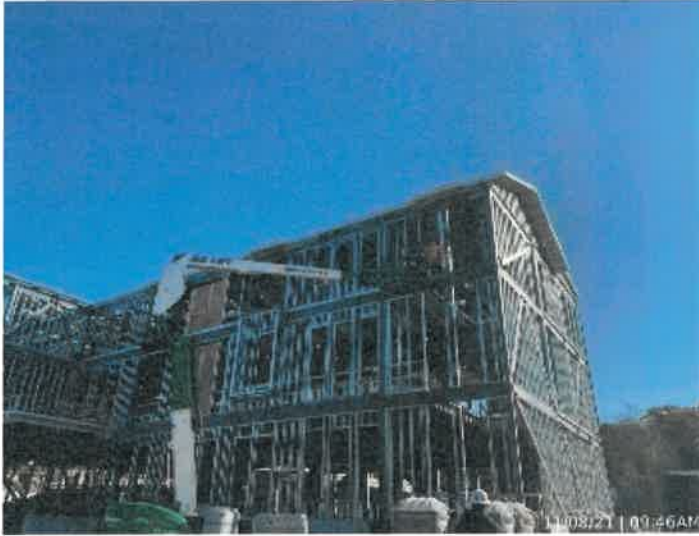
Photo depicts the progress of truss decking and framing.
