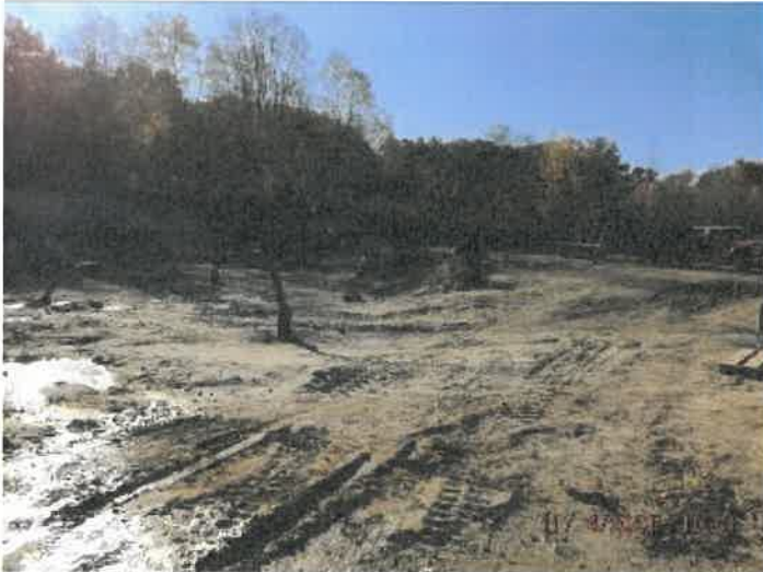
Photo depicts the progress of the geothermal wells.
