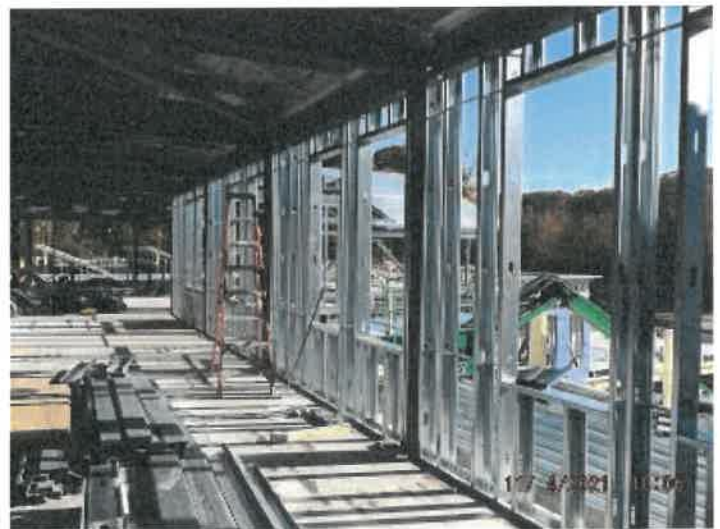
Photo depicts the progress of the third floor framing.
