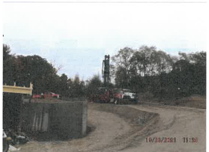
Photo depicts the progress of geothermal wells.
