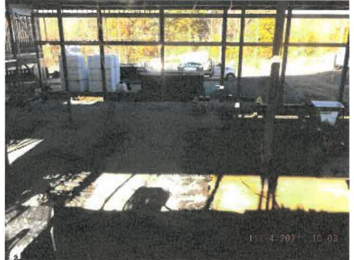
Photo depicts the overall apparatus bay progress.
