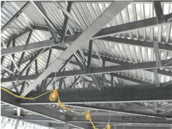
Photo depicts the progress of truss decking at the roof level.
