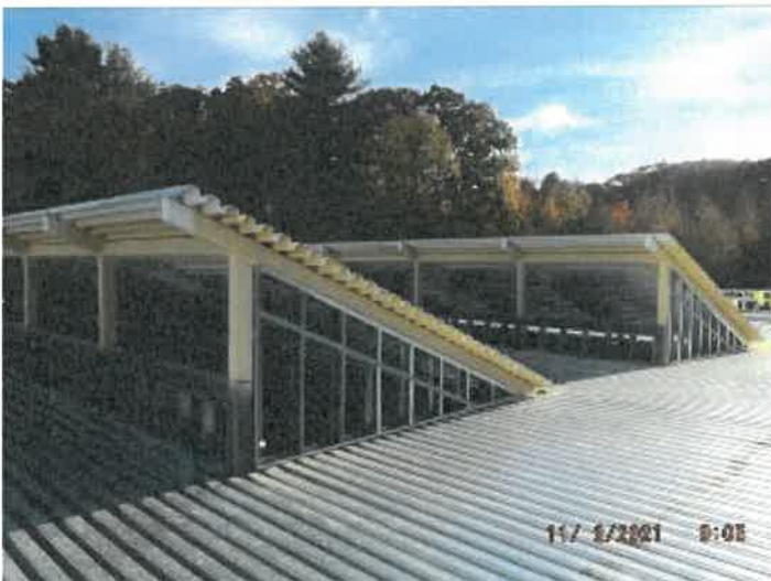
Photo depicts progress of the insulative coating.
