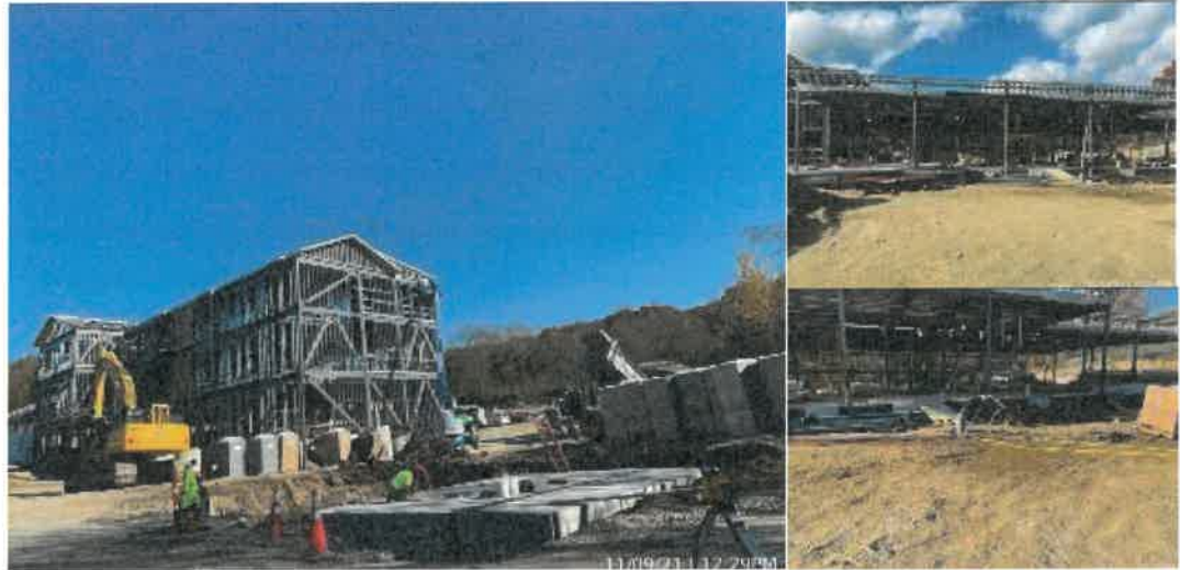
Pictures: Overall Site Progress
