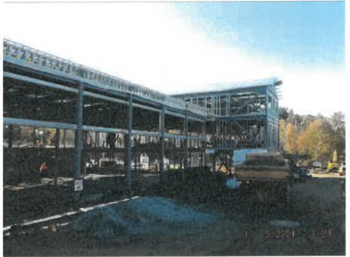
Photo depicts the progress of truss decking and parapet framing.
