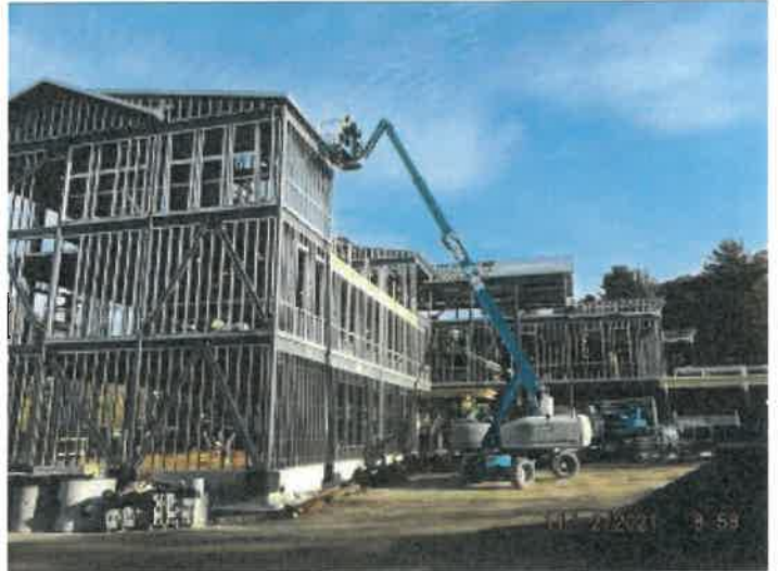
Photo depicts the progress of truss decking and framing.
