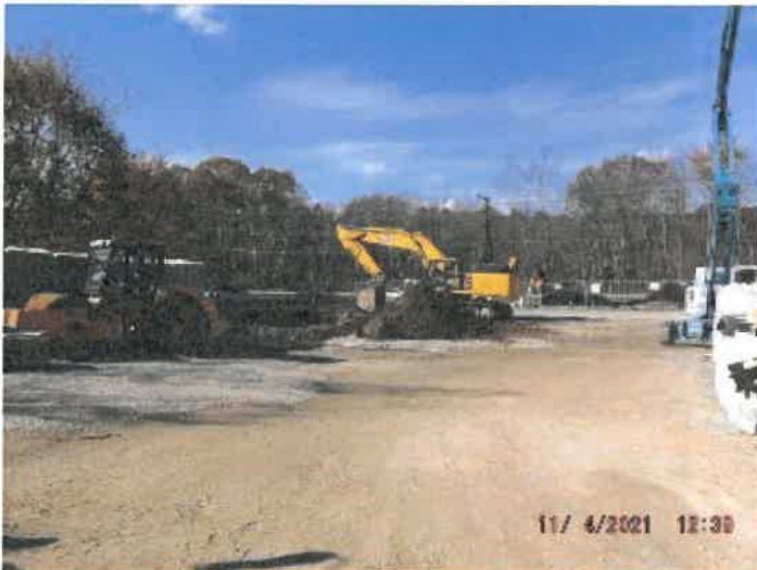
Photo depicts the progress of site drainage structures and piping.
