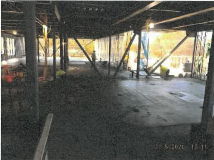
Photo depicts the progress of the slab on grade.
