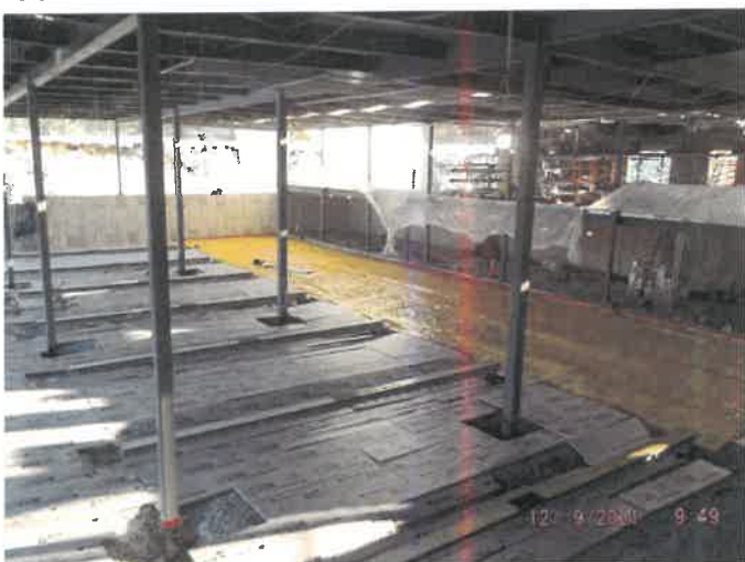
Photo depicts progress of the Apparatus bay slab prep.
