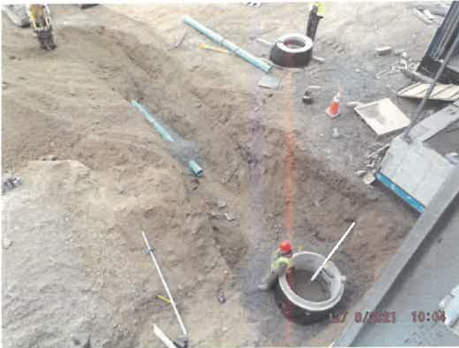
Photo depicts the progress of the underground utilities and drainage.
