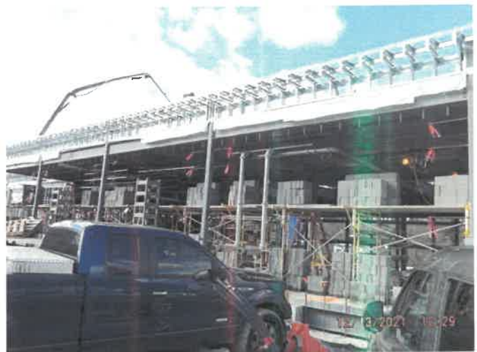
Photo depicts the progress of the parapet framing and CMU installation.
