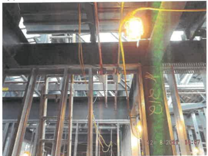
Photo depicts the progress of truss decking and HVAC piping.
