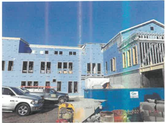
Photo depicts the progress of the exterior sheathing and blocking.
