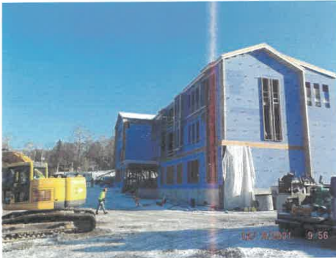
Photo depicts the progress of the exterior sheathing and blocking.
