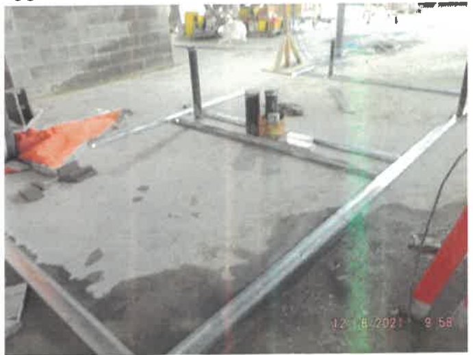
Photo depicts the progress of the first floor framing.
