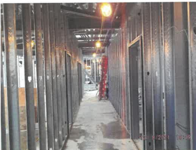
Photo depicts the progress of second floor framing.
