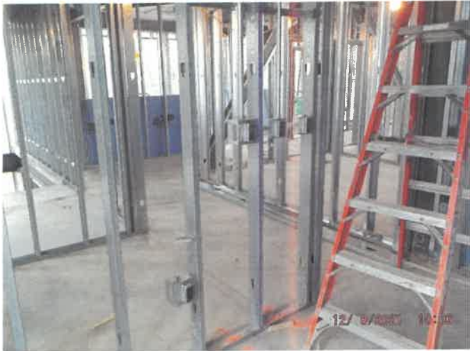
Photo depicts the progress of the third floor electrical rough-in
