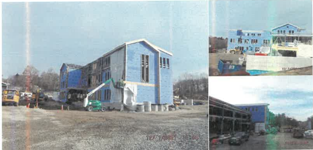
Pictures: Overall Site Progress
