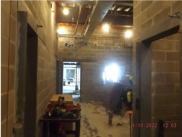
Photo depicts the progress of the detention area.
