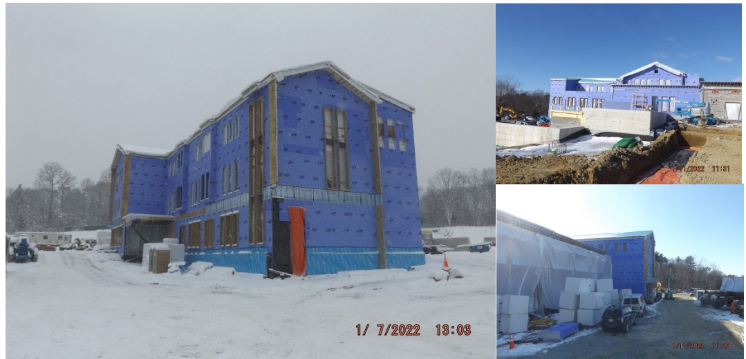
Pictures: Overall Site Progress
