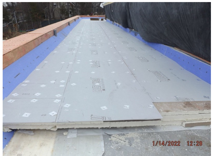
Photo depicts the progress of the apparatus bay roof.
