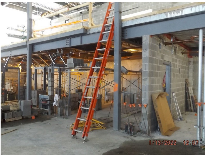
Photo depicts progress of the Apparatus bay support rooms.
