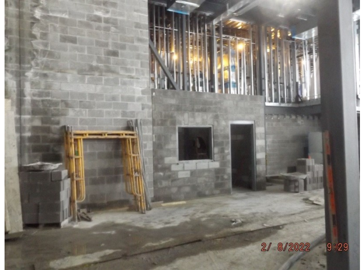
Photo depicts the progress of the apparatus bay and watch room.
