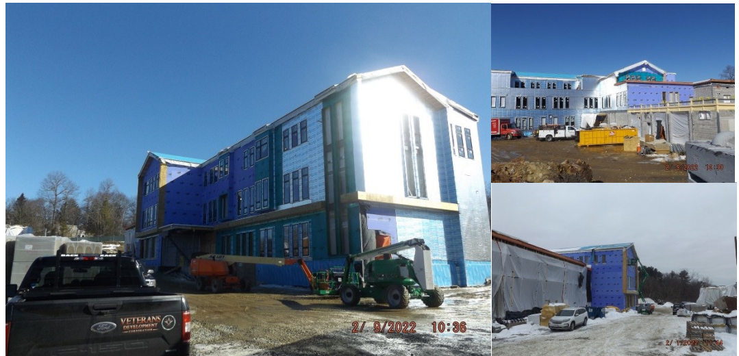
Pictures: Overall Site Progress
