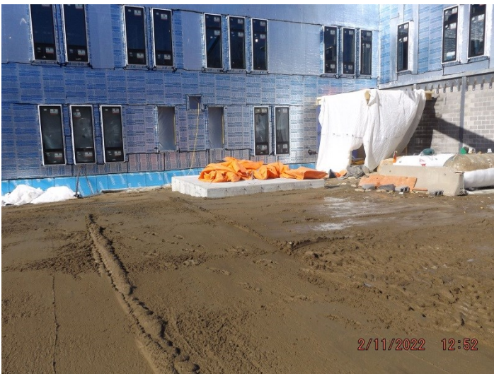
Photo depicts the progress of the antenna tower pad.
