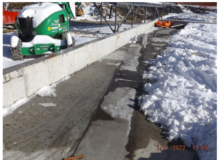
Photo depicts the progress of the second floor green roof.
