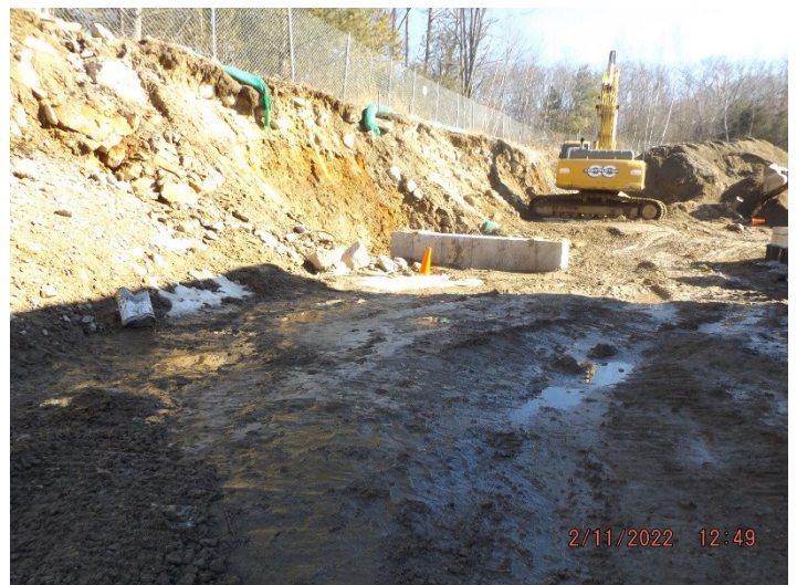
Photo depicts the progress of shooting range footings.
