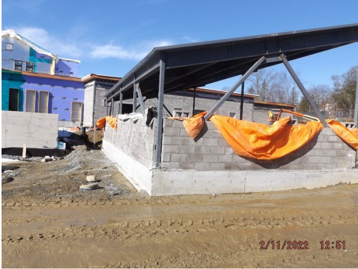
Photo depicts the progress of the carport.
