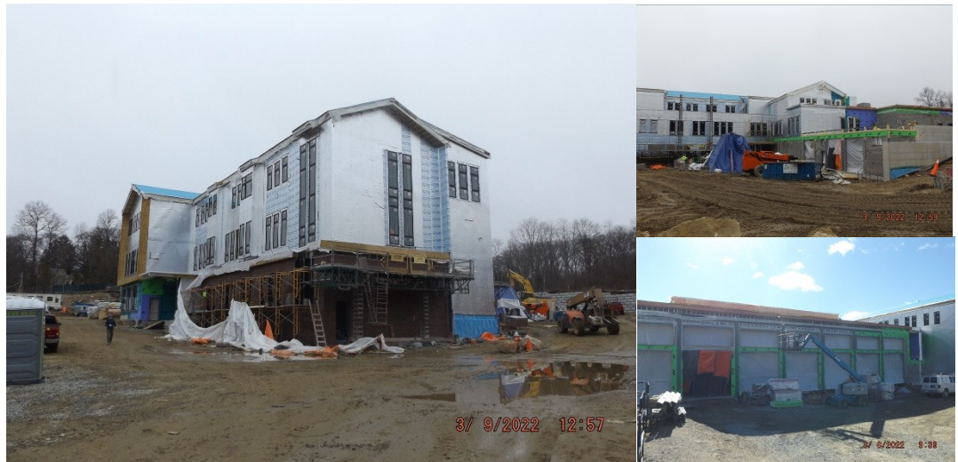
Pictures: Overall Site Progress
