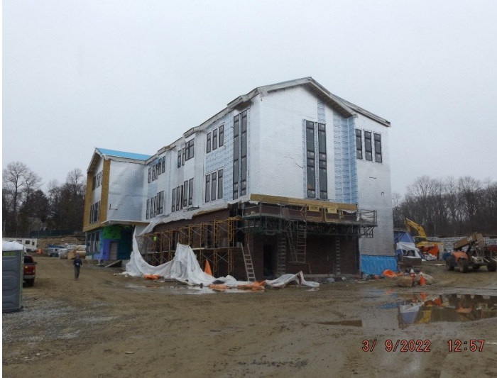
Photo depicts the progress of the AVB, window installation and brick.
