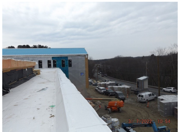
Photo depicts the progress the roof AVB and front of site.
