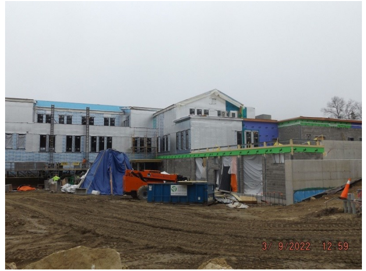
Photo depicts the progress of the AVB, framing and window installation.
