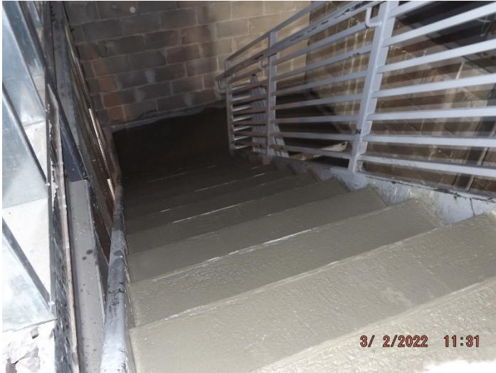
Photo depicts the Concrete for stair 1.
