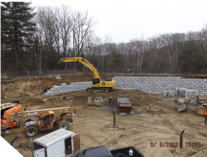
Photo depicts the progress of the retaining wall.
