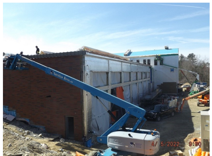
Photo depicts the progress of the AVB at the apparatus bay and metal roof soffit.
