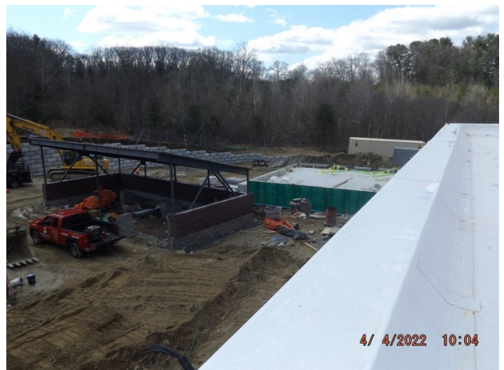
Photo depicts the progress the rear of site.
