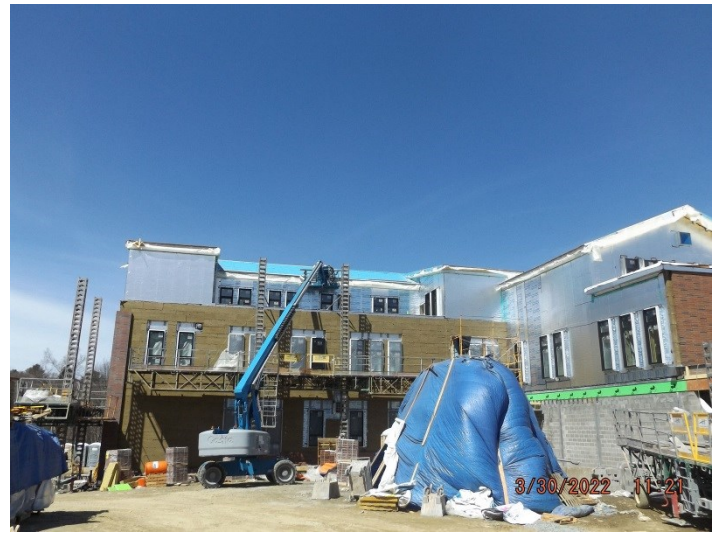
Photo depicts the progress of the AVB, framing, window installation, window trim and brick.
