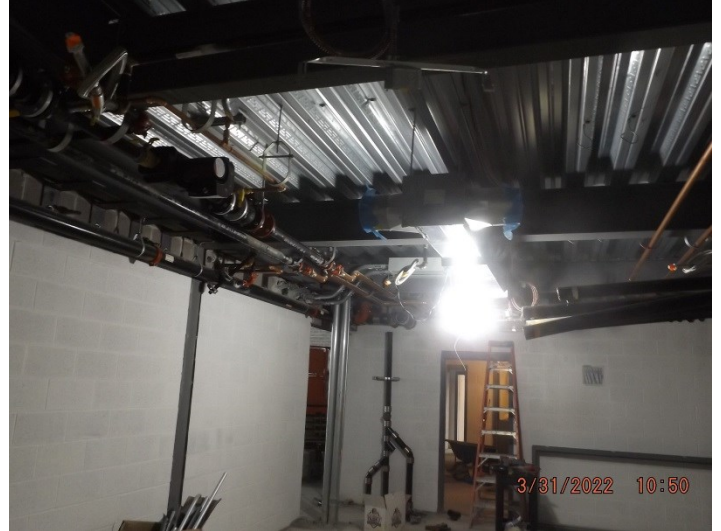
Photo depicts the progress of block-filler in the apparatus support room area.
