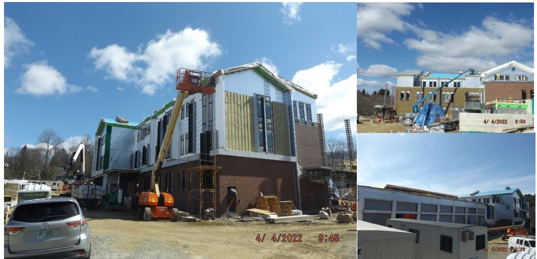
Pictures: Overall Site Progress
