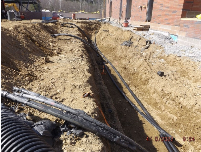
Photo depicts the progress of tying in the geo-thermal wells.
