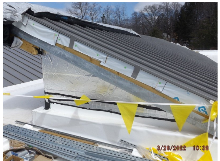
Photo depicts the progress of the metal at sawtooth roofs on the apparatus bay.
