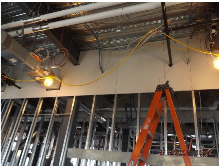
Photo depicts the progress of First floor drywall, insulated plumbing and HVAC piping and sprinkler heads.
