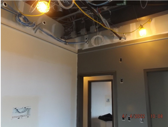
Photo depicts the progress of the third floor finishes—Paint and ceiling grid.
