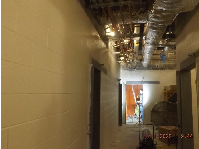
Photo depicts the block-filler in the detention area.
