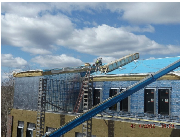
Photo depicts progress of the metal roof on the admin side.
