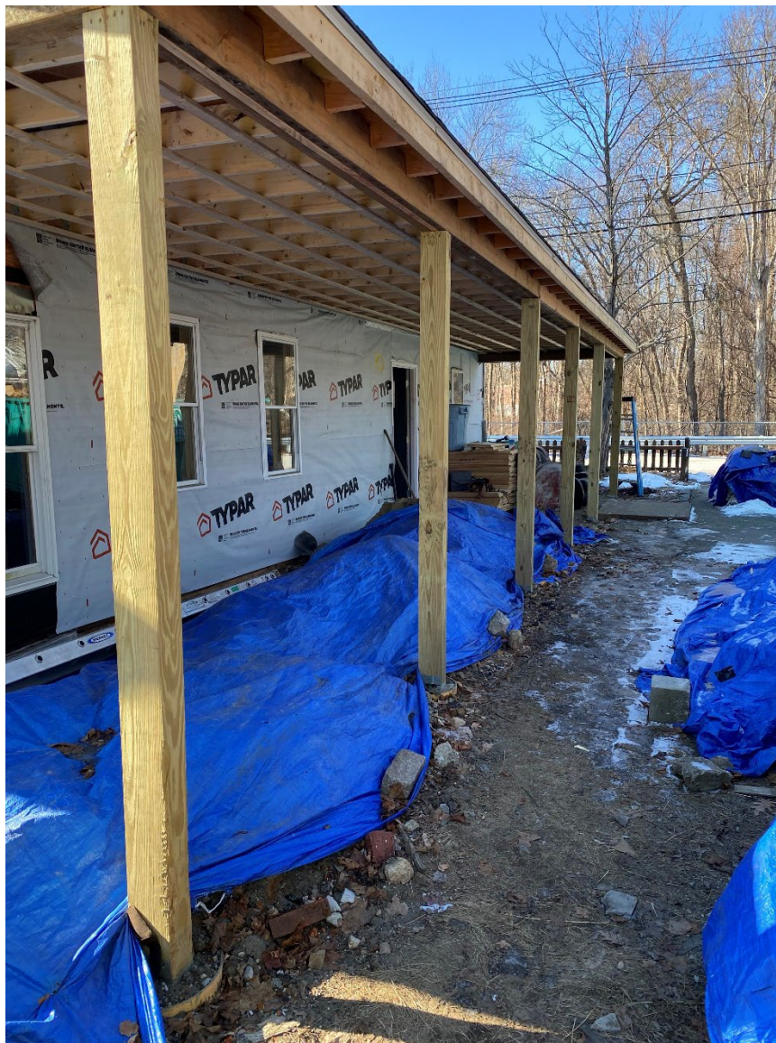
Photograph 2: View of new porch and soil stockpile, looking west.
