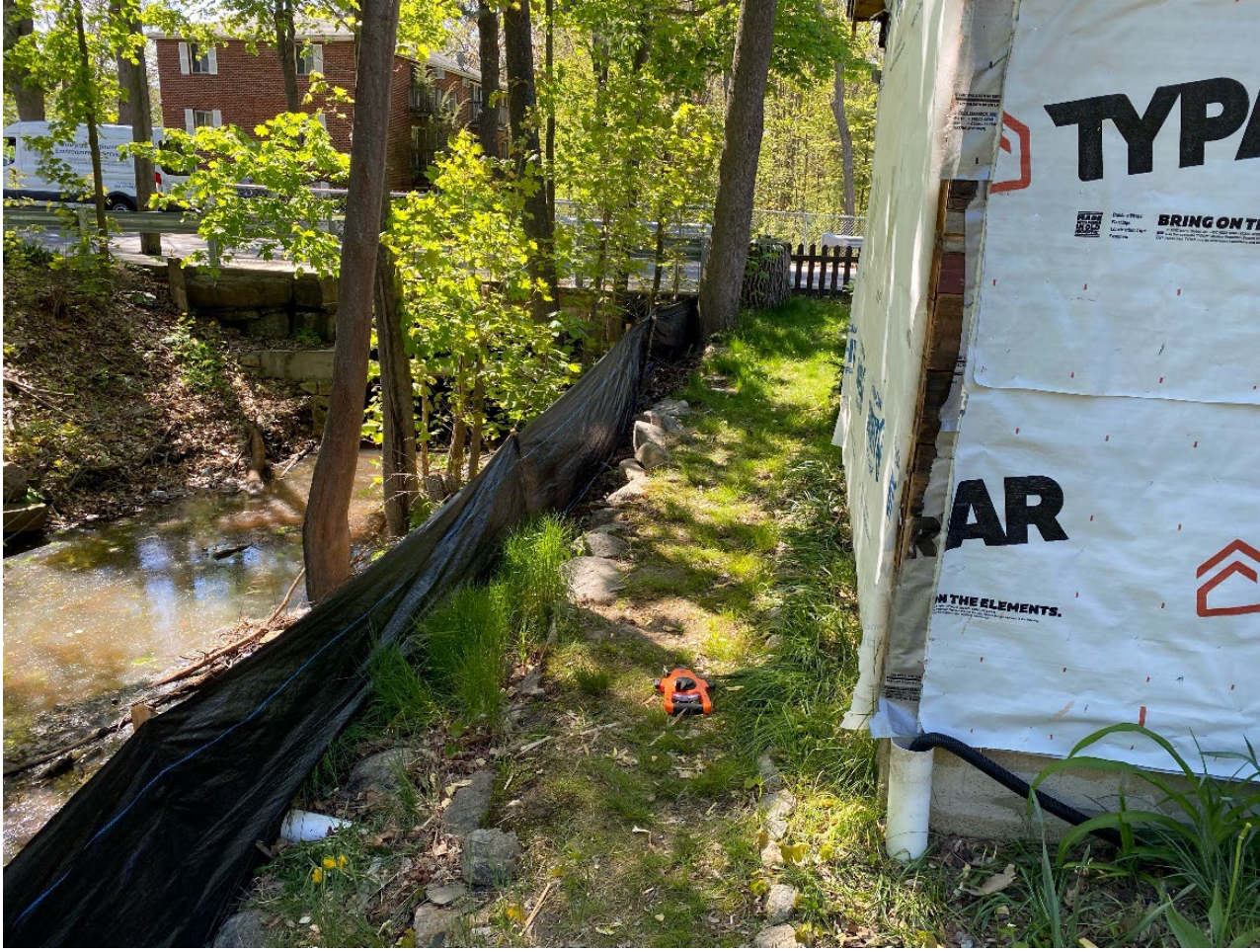
Photograph 1: PVC pipe located at the southeastern house corner, looking west.
