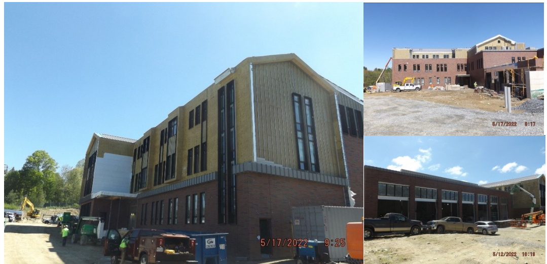
Pictures: Overall Site Progress
