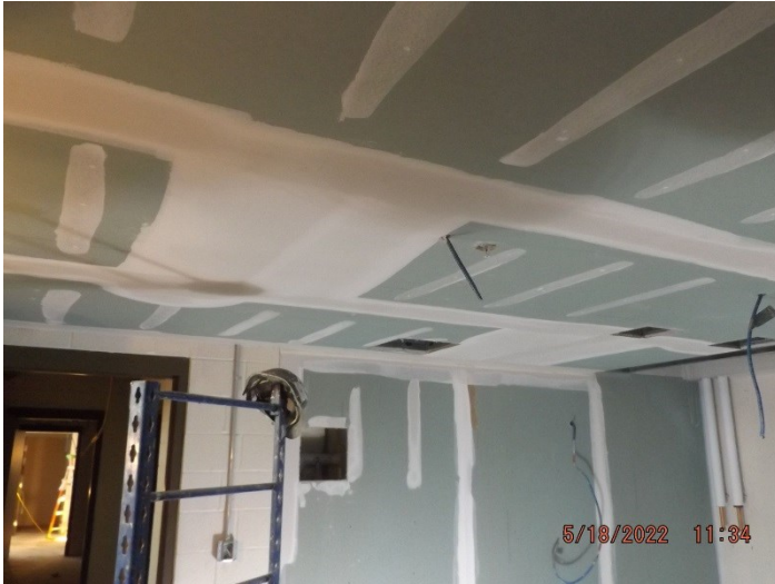
Photo depicts the progress of the apparatus support rooms.
