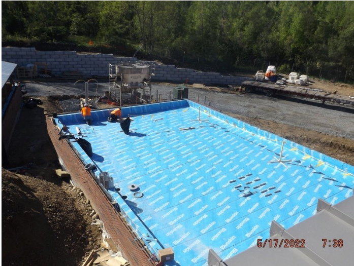
Photo depicts the progress of the lower green roof.
