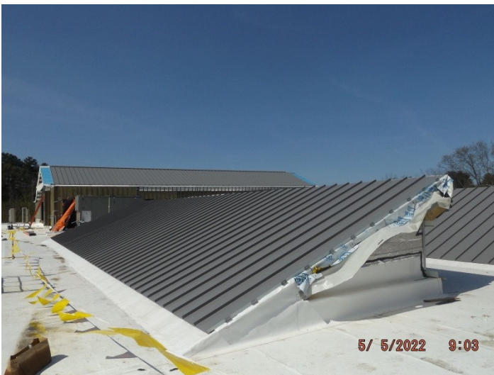
Photo depicts progress of the metal roof.
