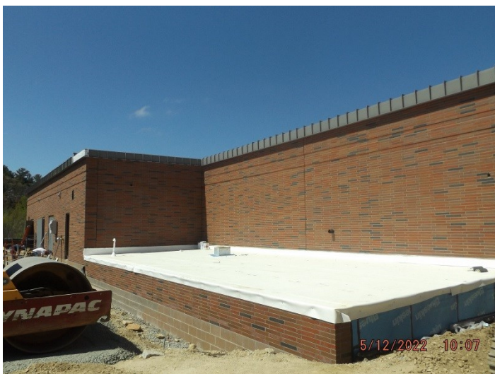
Photo depicts the progress of brick, lower roof and parapet metal.
